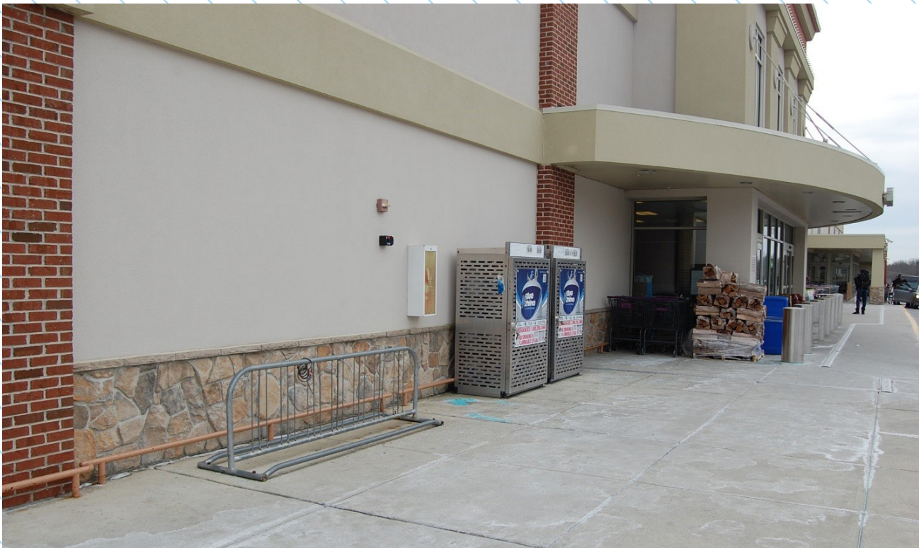
“Wheel-bender” bicycles rack, such as this in Aspen Hill, are substandard
