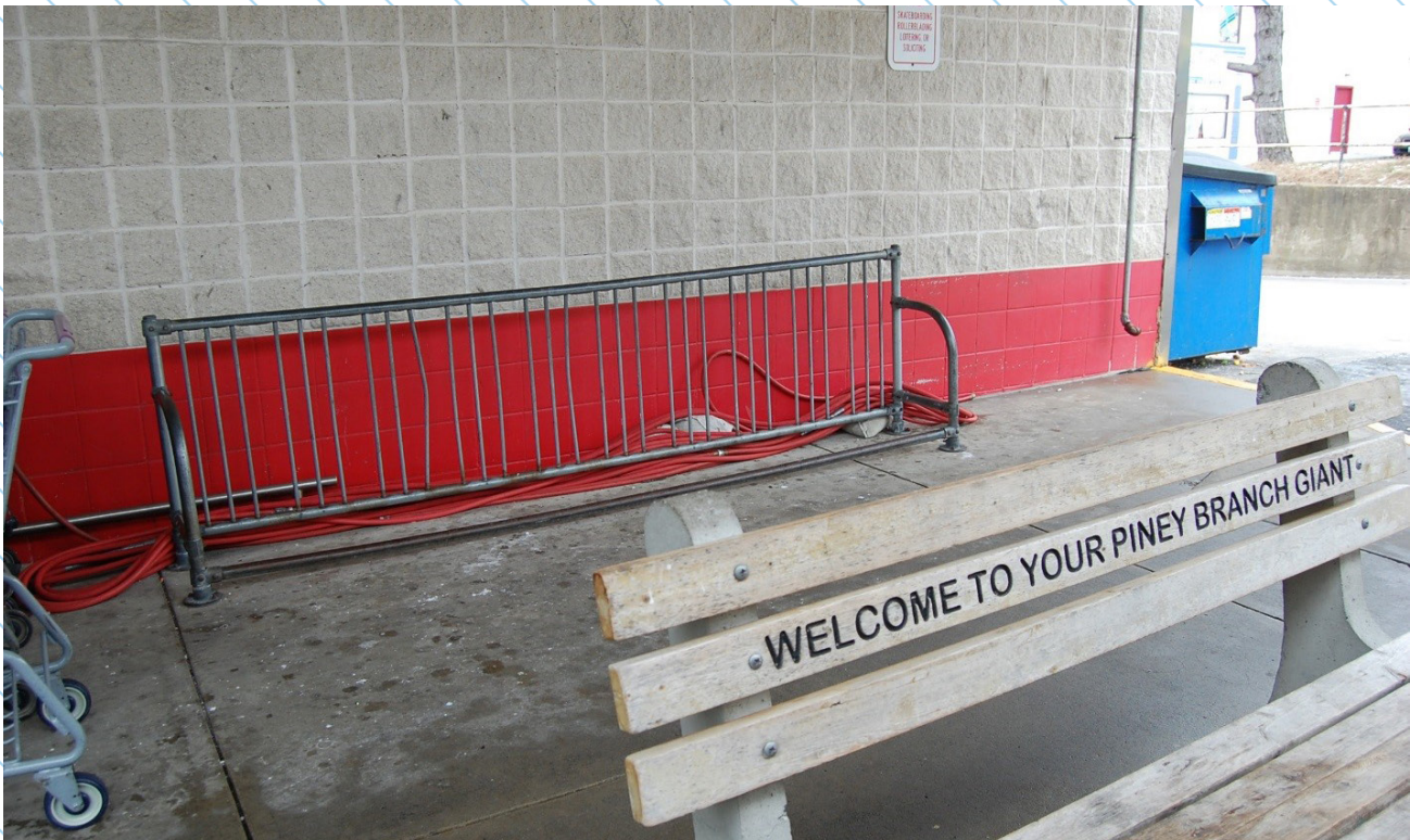
Improperly installed bicycle racks limit use
