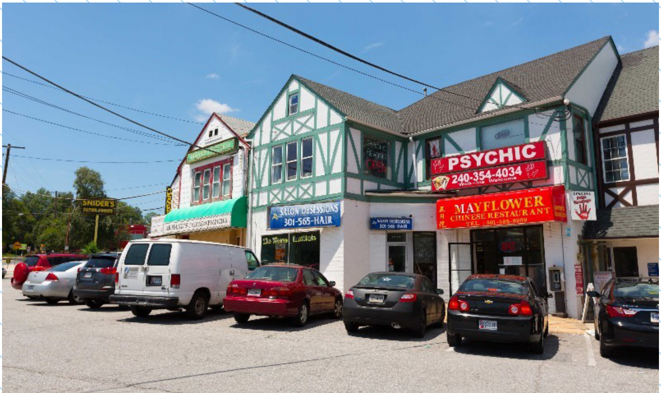
The retail areas in Montgomery Hills lack bicycle parking
