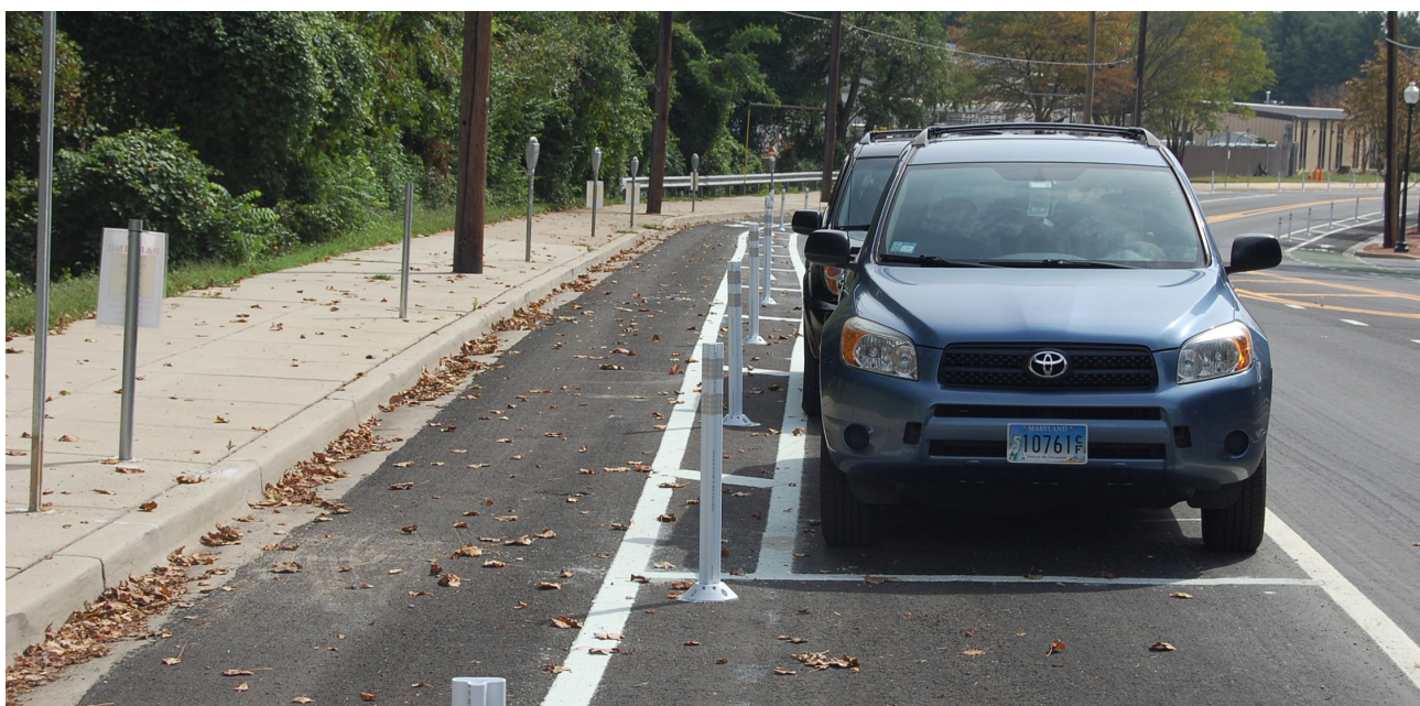
Interim separated bike lanes on Nebel Street in White Flint can be upgraded over time by development approvals or county projects
