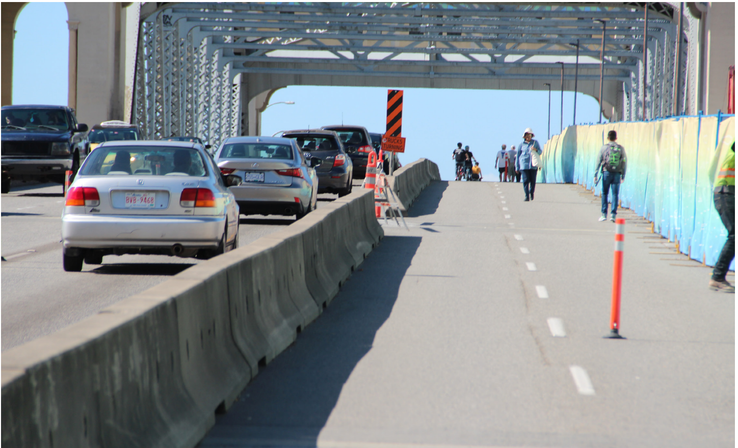
Concrete barriers provide separation from traffic on this bike lane in Vancouver, British Columbia.
