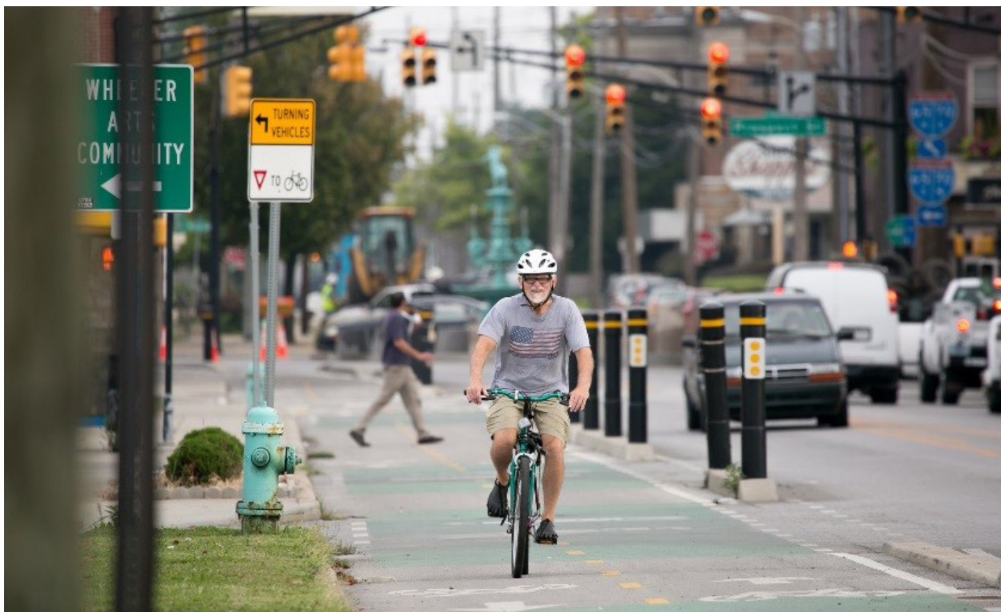
Rigid bollards with curbs provide separation from traffic for these bike lanes. Source: People for Bikes
