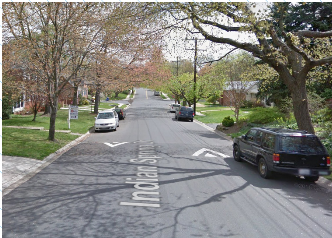
Un-laned, two-way “yield” streets, such as Indian Spring Drive, are common in residential neighborhoods in Montgomery County
