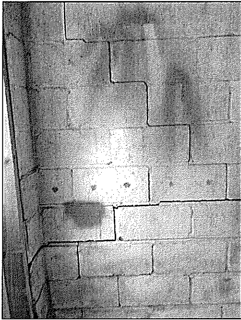
Figure 2: Interior of garage showing cracking in masonry
