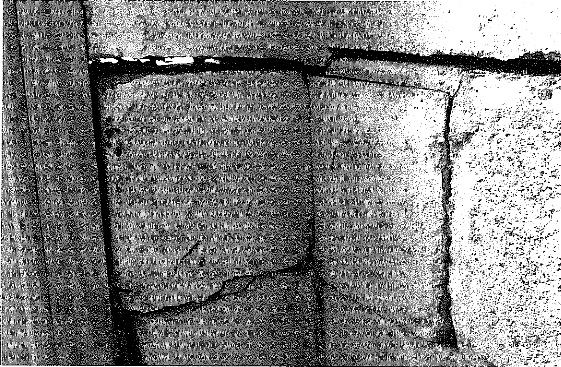
Detail: 7304 Willow Ave., Garage wall crack detail
