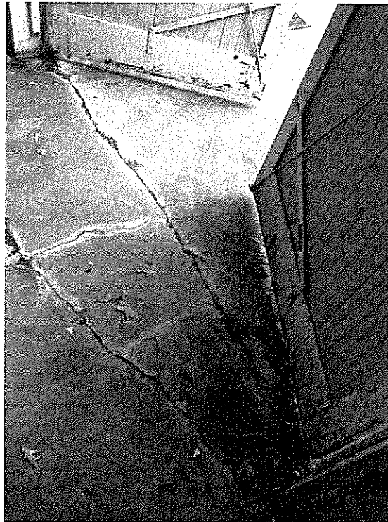
Detail: 7304 Willow Ave., Garage wall floor slab/ root heave
