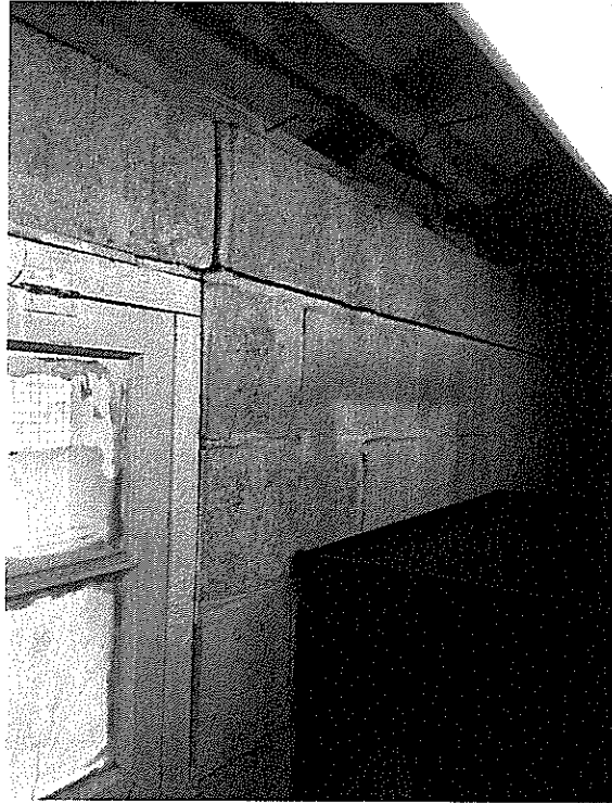
Detail: 7304 Willow Ave., Garage wall crack high
