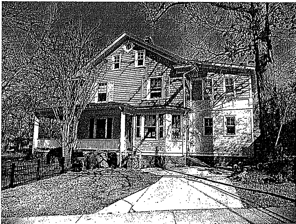
COMPLETE SIDE VIEW (ALONG COLUMBIA AVE.)
