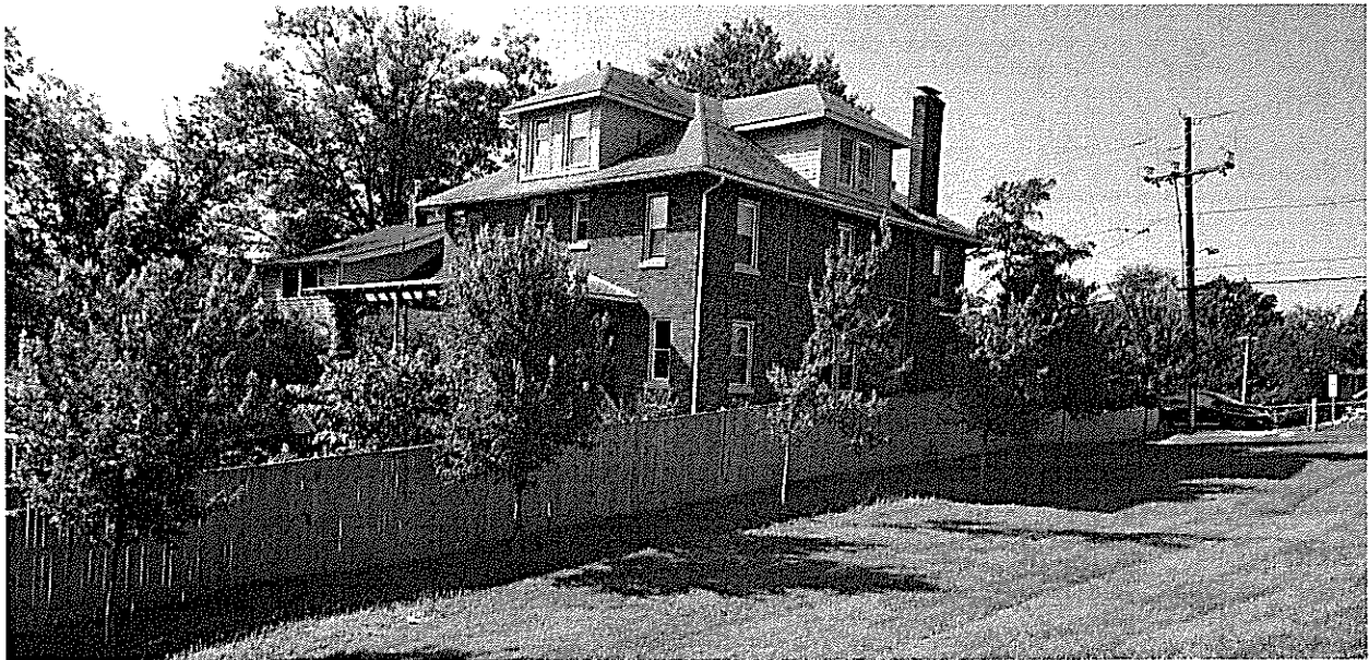
Figure 2: The subject fence looking southeast.
