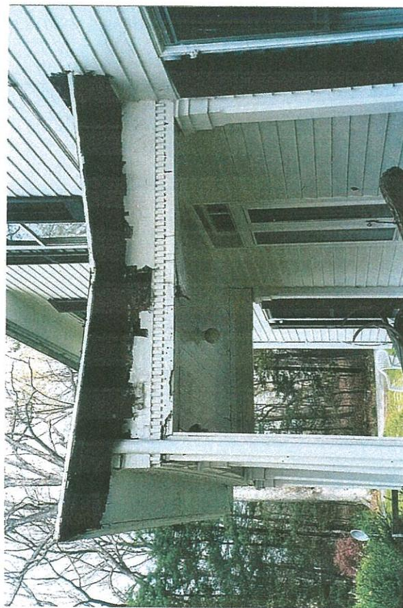
Photographs from 2007 showing clearly degraded roof and overhang and the location of the single downspout at the southeast post.
