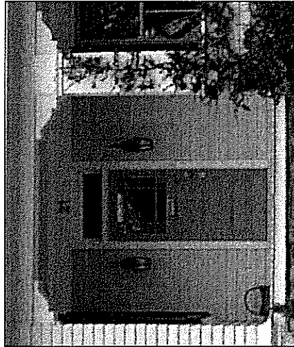
Brackets, including knee braces and exposed rafter tails are typical Craftsman style building elements. (Takoma Park, MD)
