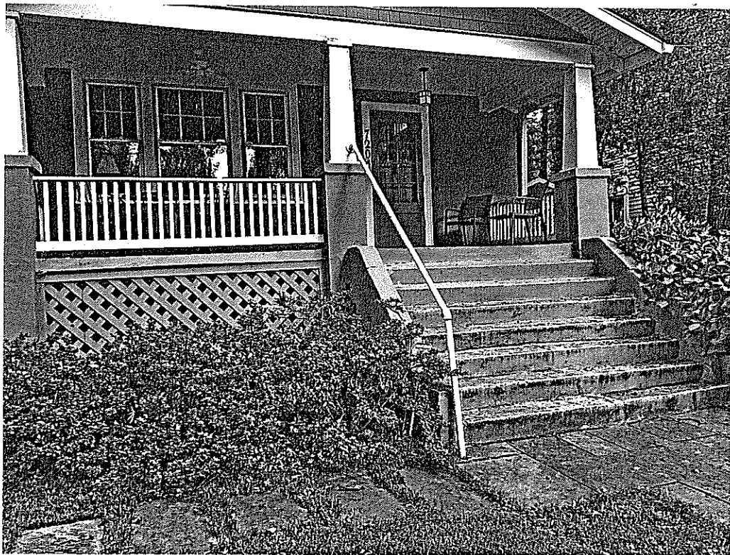
FRONT PORCH + STEPS
