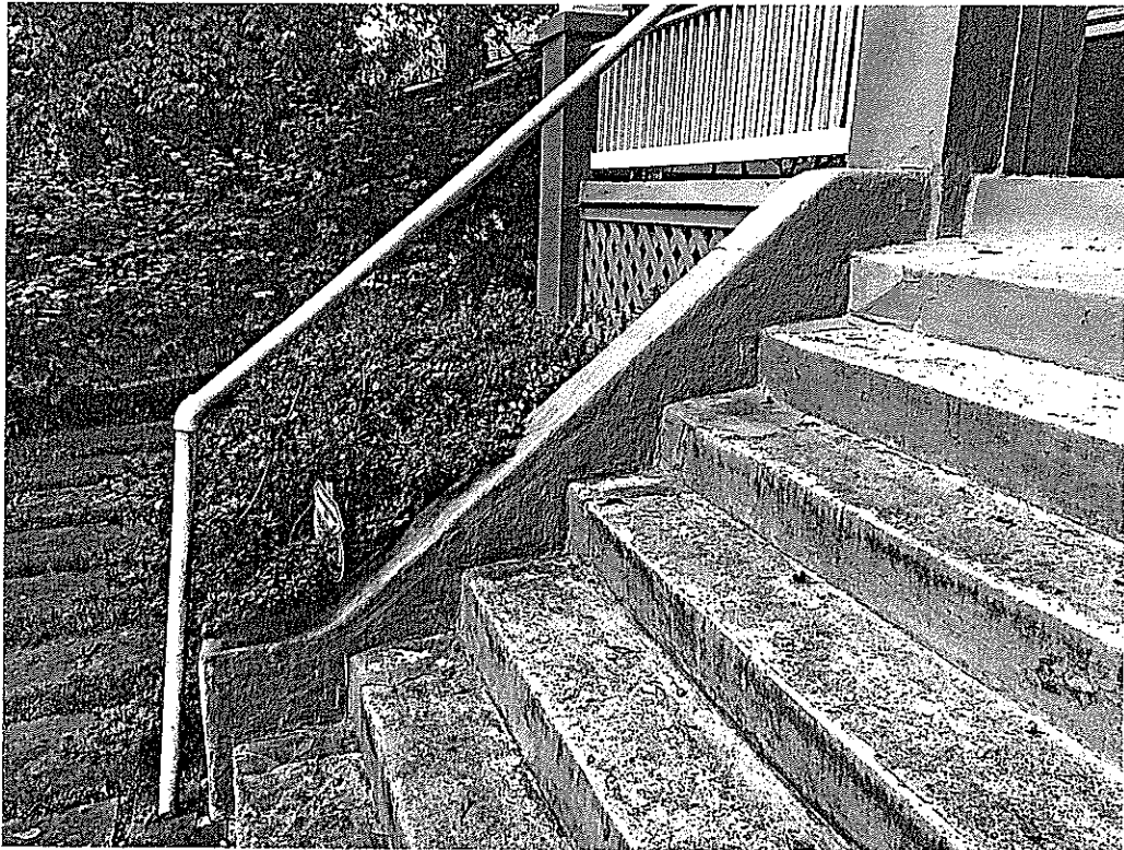
CONCRETE STEPS W/ PIPE RAIL
