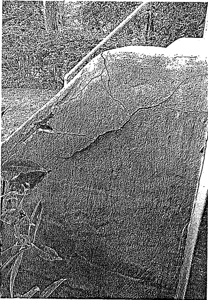
DAMAGED SIDE WALL
