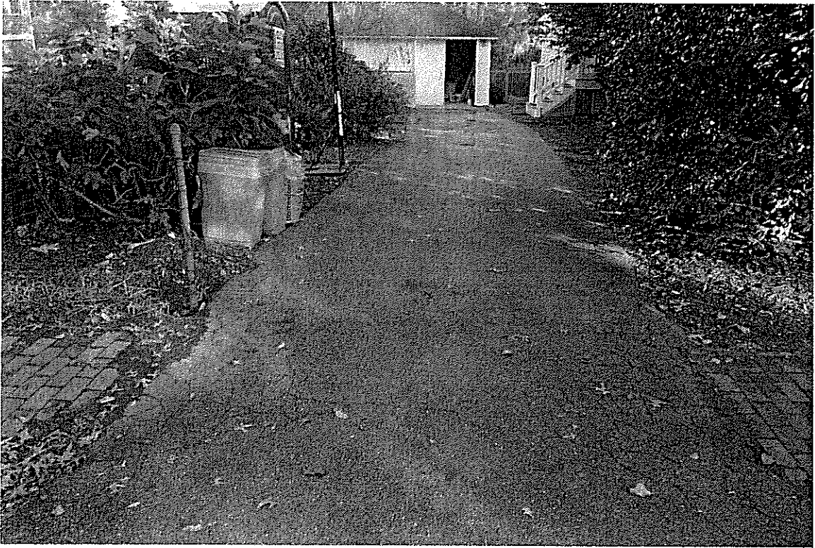
Existing driveway from public right of way.
