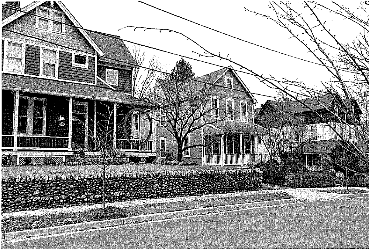
Figure 1: The proposals is to replace the circled window.
