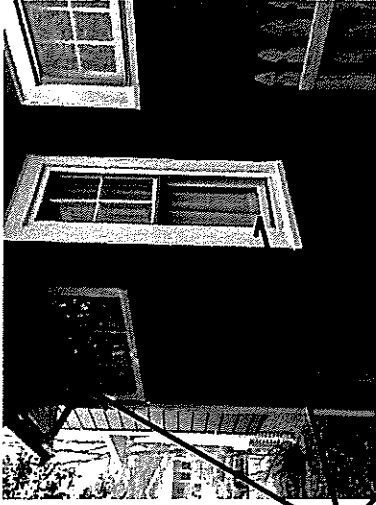
Rear of Bay
