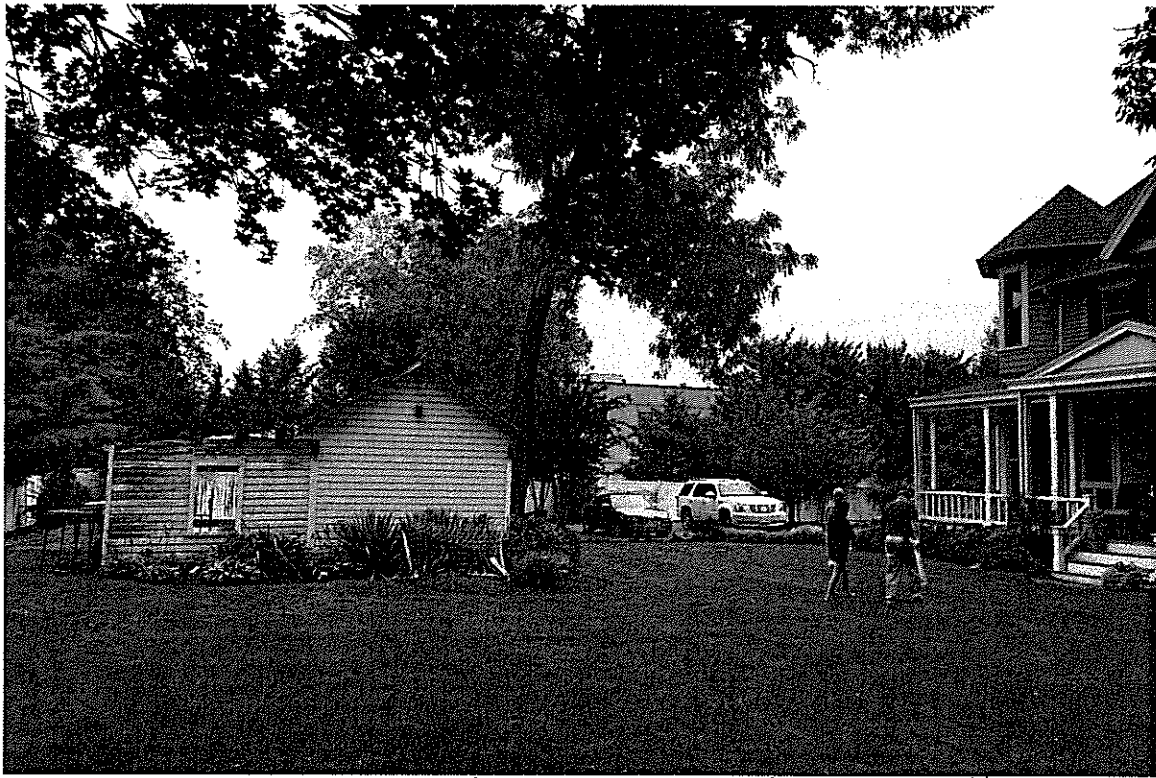
LEFT SIDE OF EXISTING SHED IN RELATION TO MAIN HOUSE
