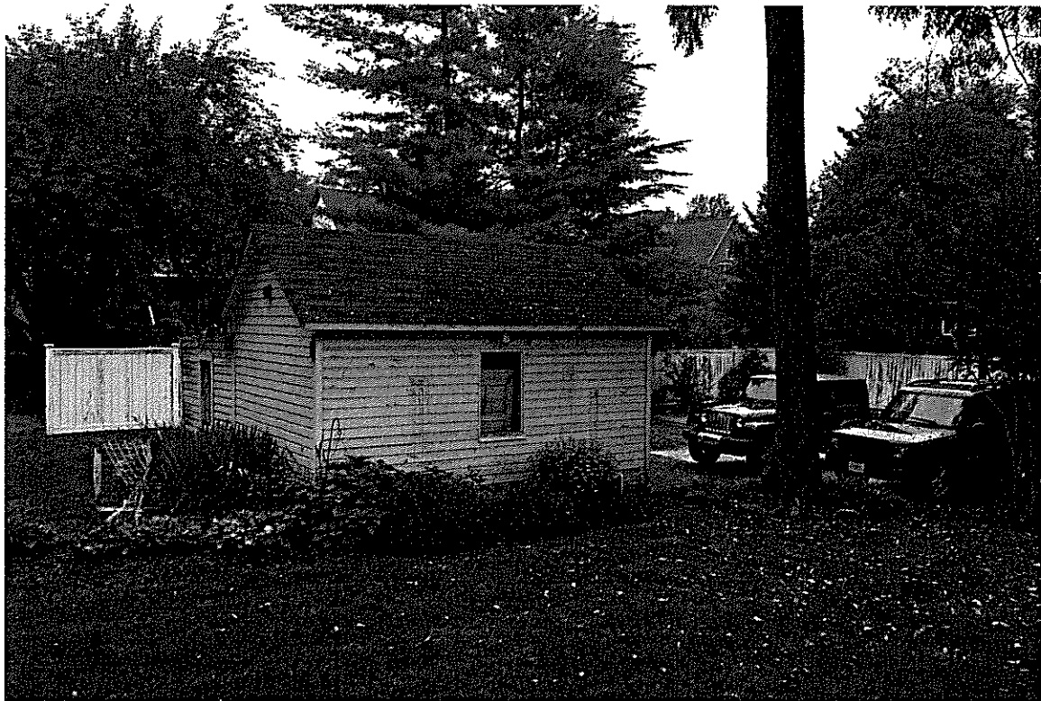
FRONT OF EXISTING SHED AND DRIVEWAY BEYOND.
