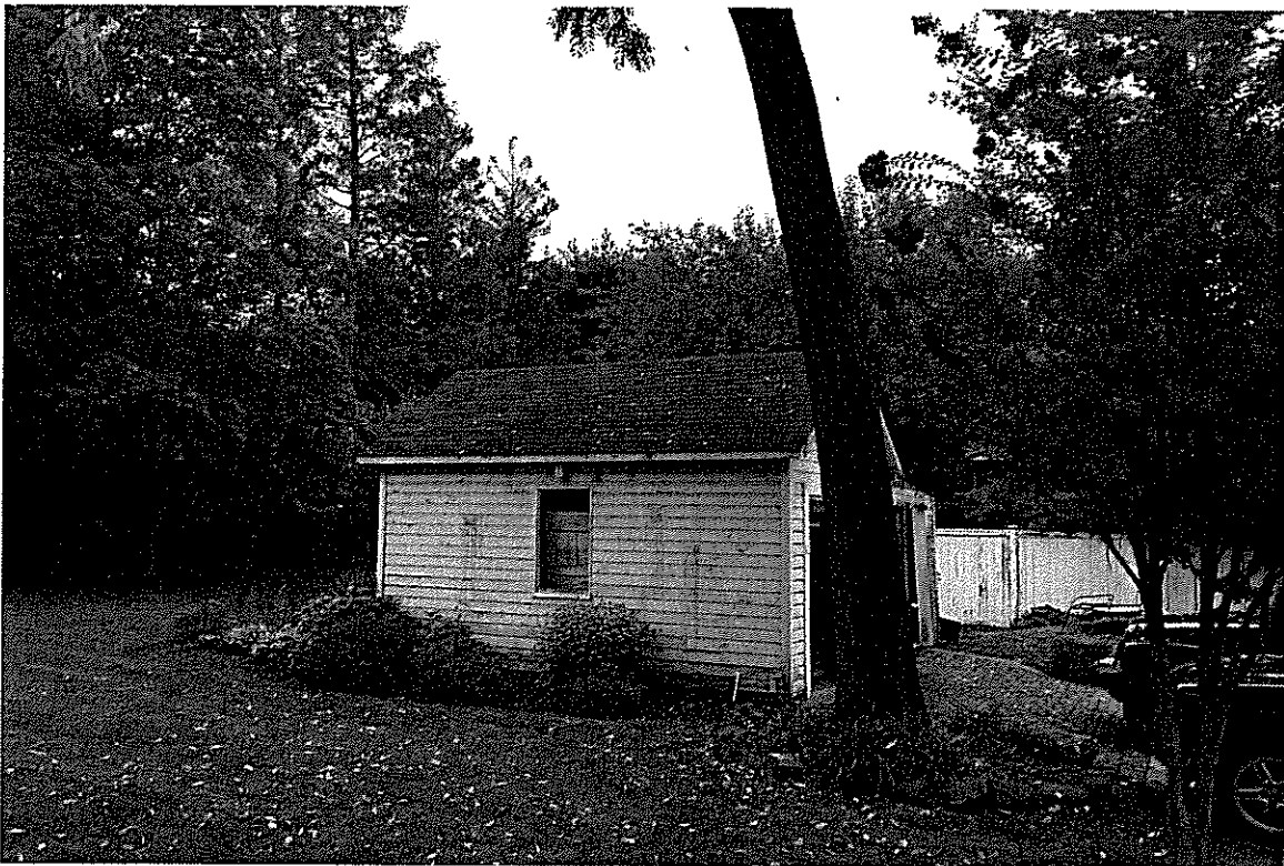
FRONT-RIGHT SIDE OF EXISTING SHED
