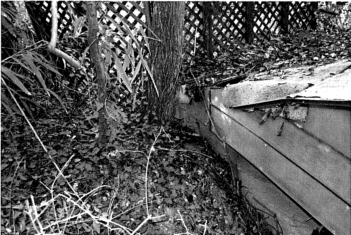
VIEW OF TREE BASE ABUTTING GARAGE
