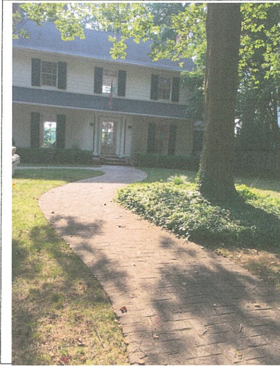
Detail: IMPERVIOUS FRONT WALK SET IN CONCRETE TO BE REPLACED WITH PA BLUESTONE SET ON DUST
