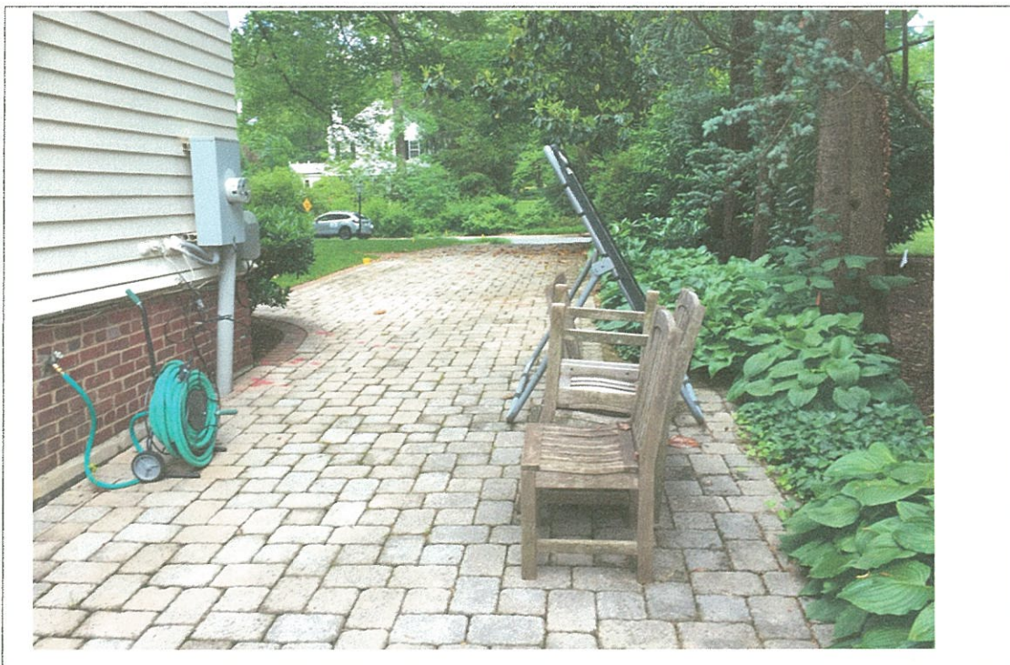
EXISTING IMPERVIOUS PAVER DRIVEWAY TO BE REMOVED AND REPLACED WITH SECTIONS OF Detail: COBBLE AND PERMEABLE GRAVEL, HISTORICALLY APPROPRIATE
