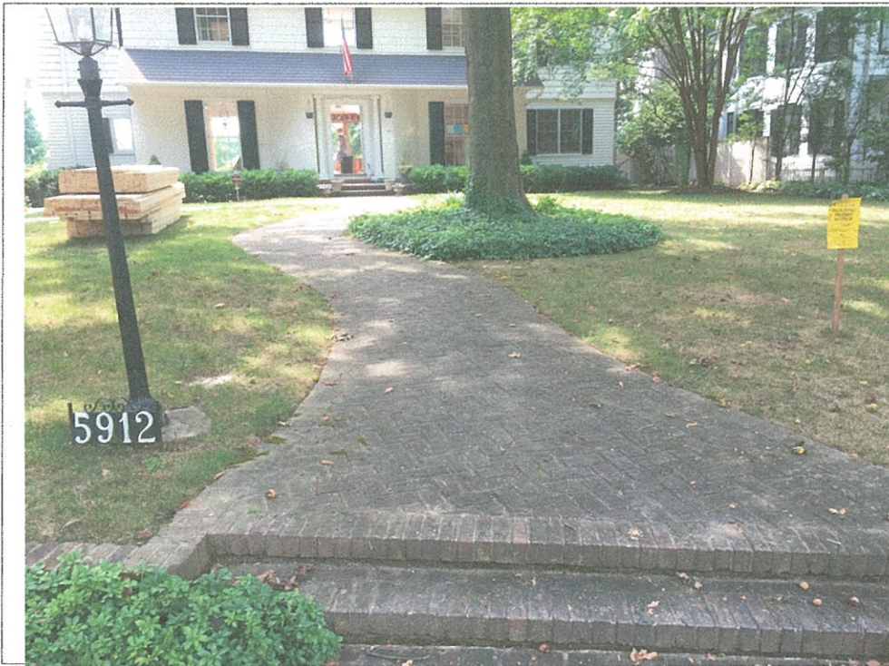
Detail: BRICK STEPS TO BE REBUILT IN LINE WITH STRAIGHT BLUESTONE FRONT WALK
