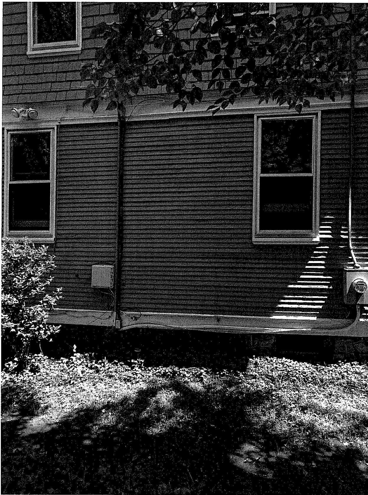
Photo of area where the door will be added.
