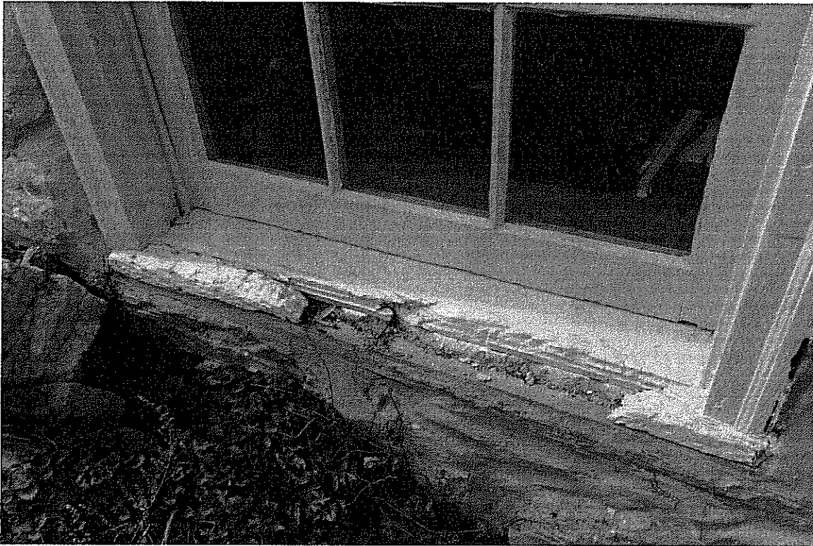
⑨ Close-Up of Rotten Sill and Trim at Existing Lower Level Window
