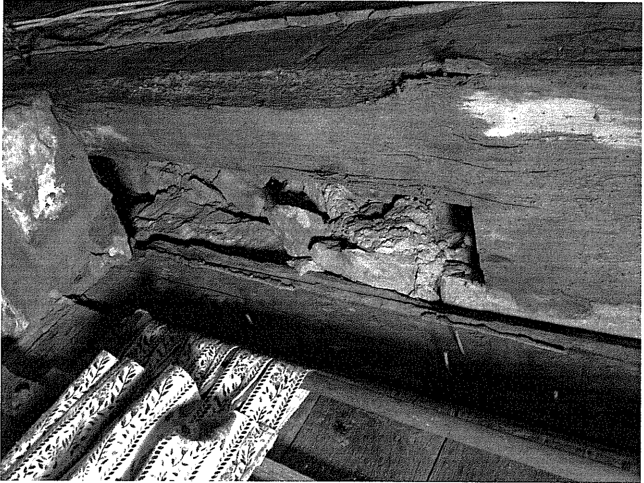
⑥ Close-Up of Wood Header with Rotten Section Removed
