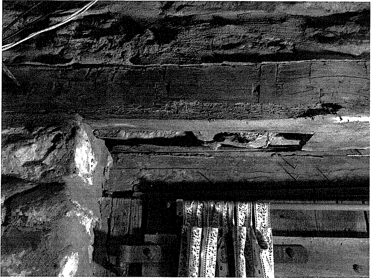
⑤ Close-Up of Rotten Wood Header
