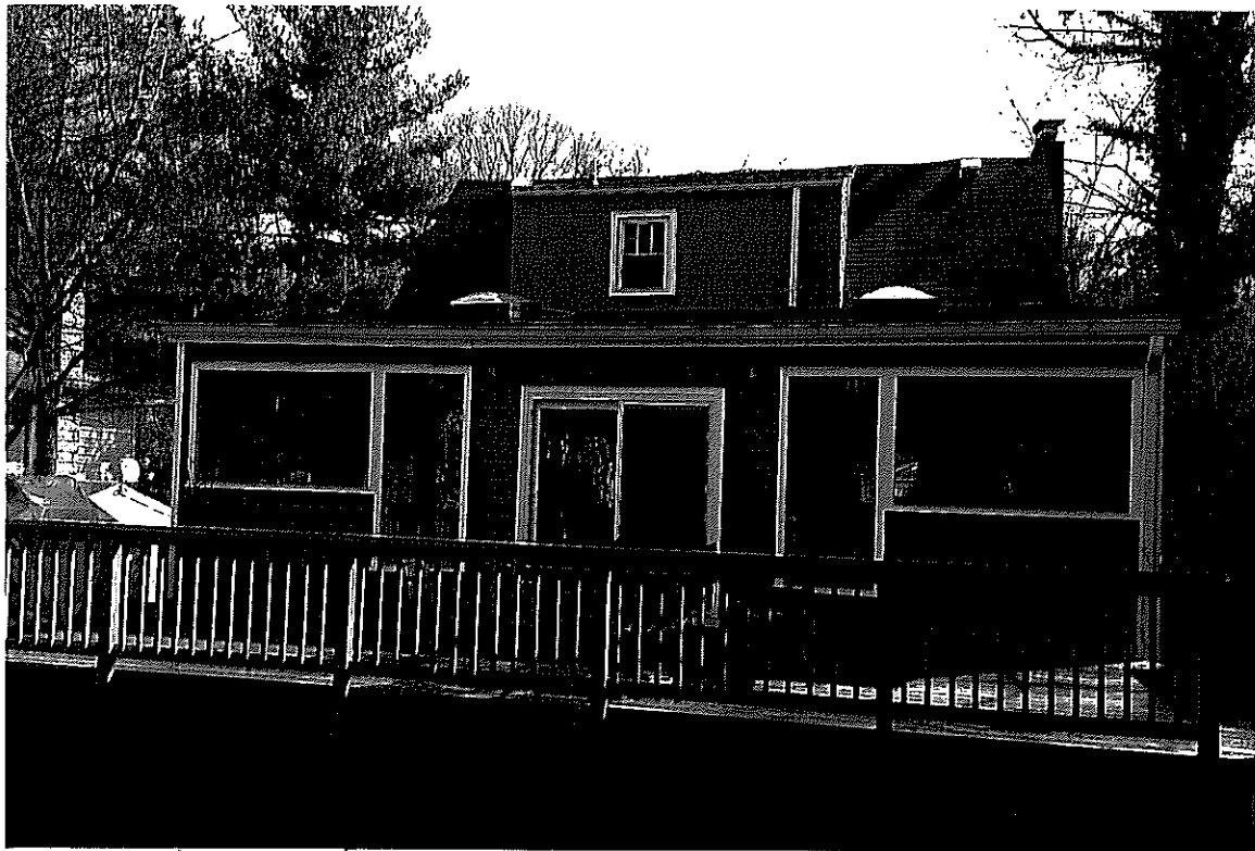
Detail: REAR of HOUSE
