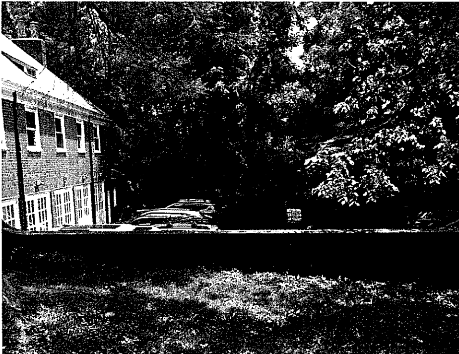
View from Lawn to Historic Wall and Teale Center
