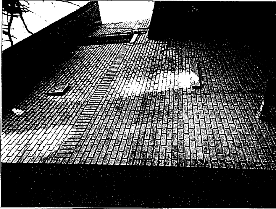
Detail: Garage rear (south)
