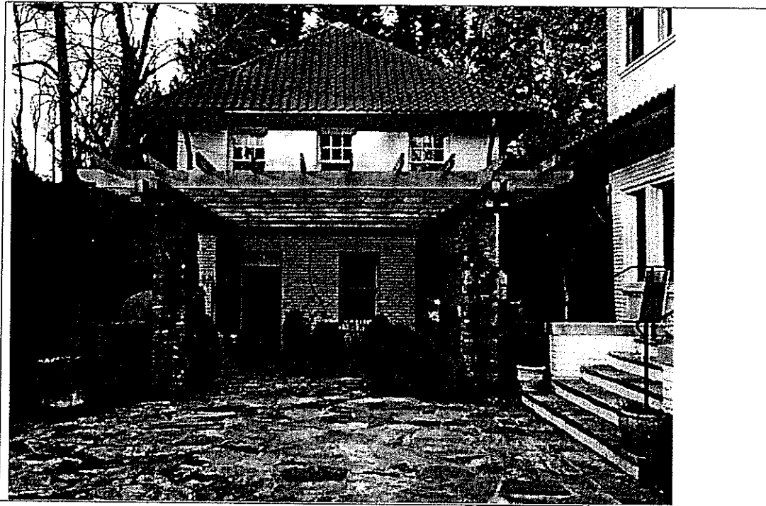
Detail: Garage from patio (east)
