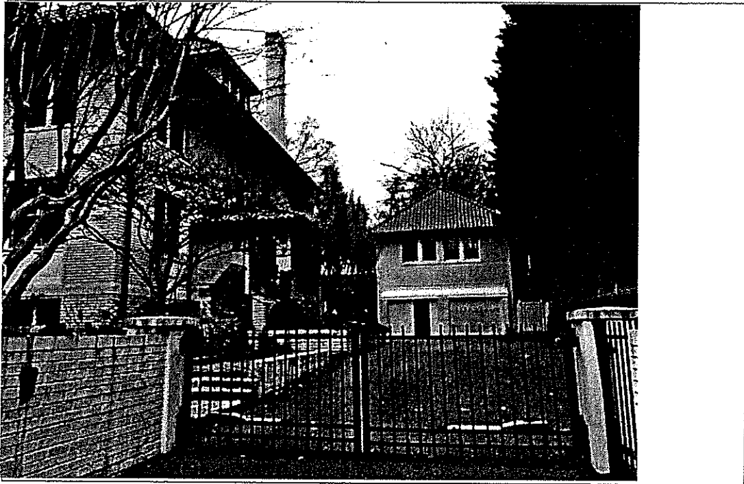
Detail: Garage from W. Irving Street (north)
