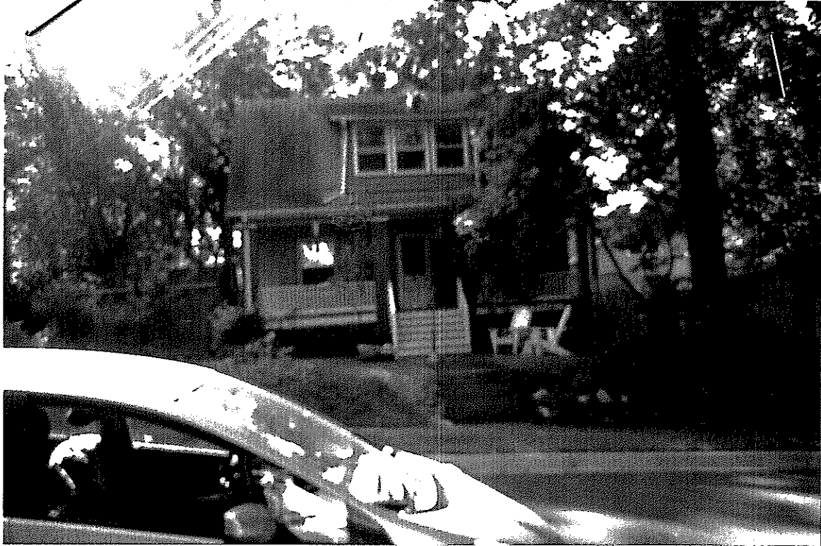
Detail: Adjacent property at 7426 Buffalo Ave
