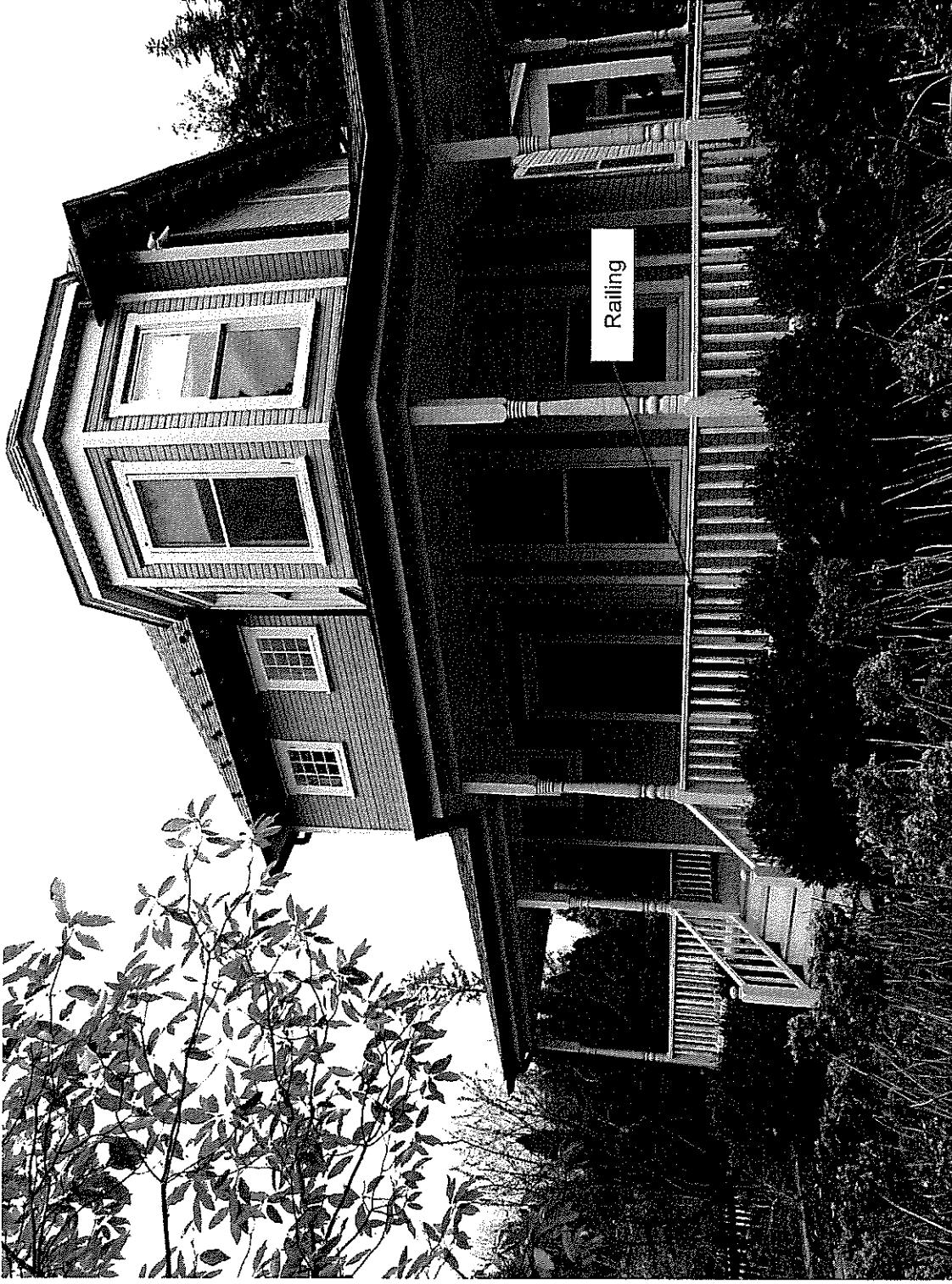
IMAGE 04c: Precedent @ 4722 Dorset: Front Elevation. Current railing replaced in-kind to match original, historic railing.
