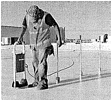
1 Simple Way to Reduce Roof Installation Costs
