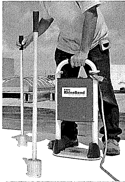
Rhinobond TPO roof system installation
