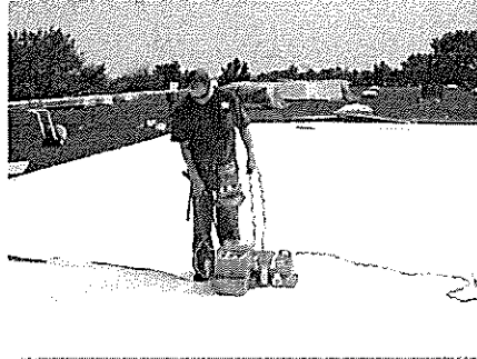
Rhinobond TPO roof system installation
