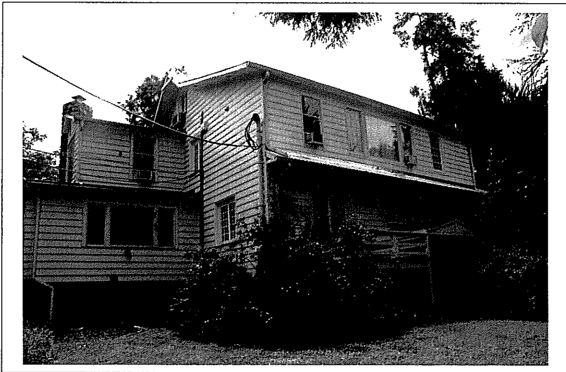
Existing West elevation. Addition to occur at this location. Dormer at second level Detail: to be reduced and original roof line at this elevation to be reconstructed.
