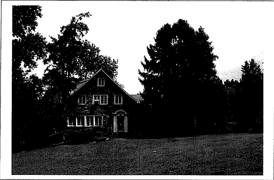
Existing South elevation. Addition to occur on left side of image (West elevation) Detail: along with extension of front patio along entire elevation.
