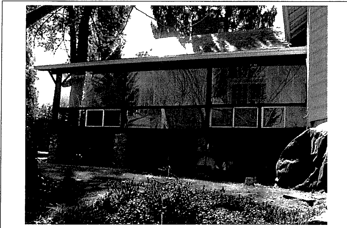
Existing North elevation. Rear porch in poor condition; plexi-glass to be replaced Detail: with insulated glazing and structure to be replaced with new posts to support roof.
