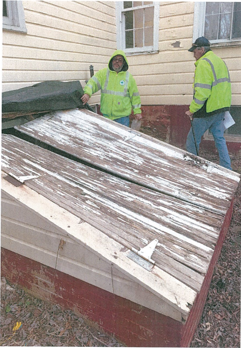
West elevation: extant deteriorated Bilco doors to be replaced.
