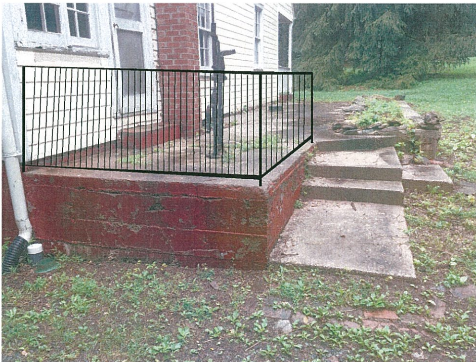
Proposed 36"-high rail photoshopped to show proposed location. It will actually end at the top of the second step rather than extend an additional 24" to the third step. This will allow users to step up toward the kitchen door without having to back track around the rail.
