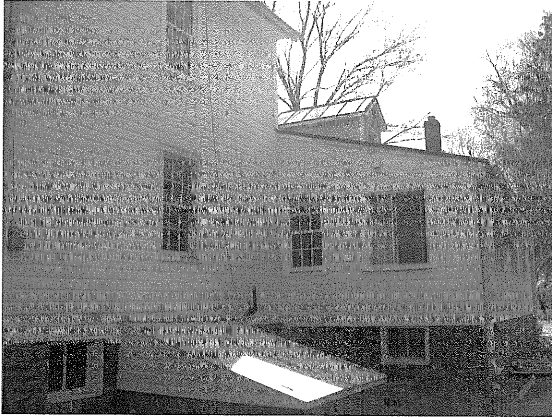
West elevation: 2009 photo showing 1950s kitchen/bathroom addition and location of basement windows. Panes to be replaced with wire mesh in window are to left of Bilco door, in the one shown at the bottom edge of the Bilco door, and in one to the far right of downspout; the latter two being part of the 1950s kitchen addition. The kitchen basement is not connected to the basement under the original portion of the house which is accessed through the Bilco doors.
