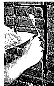
This mortar is the proper consistency for repointing historic brick. Photo: John P. Spewick.
