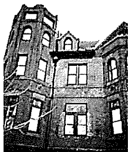
Unskilled repointing has negatively impacted the character of this late-19th century building. Photo: NPS files.
