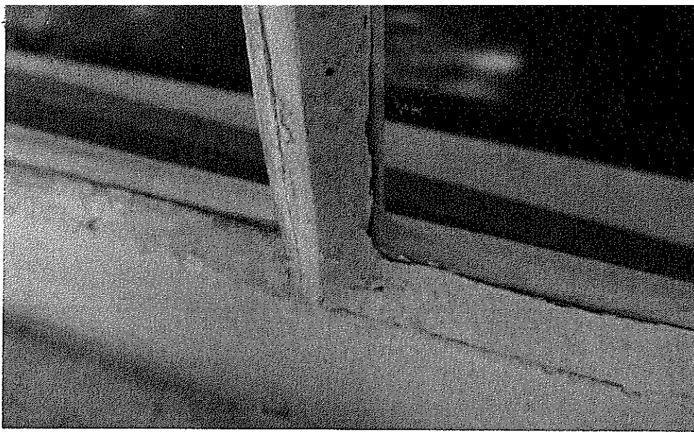
Original window requiring painting and glazing
