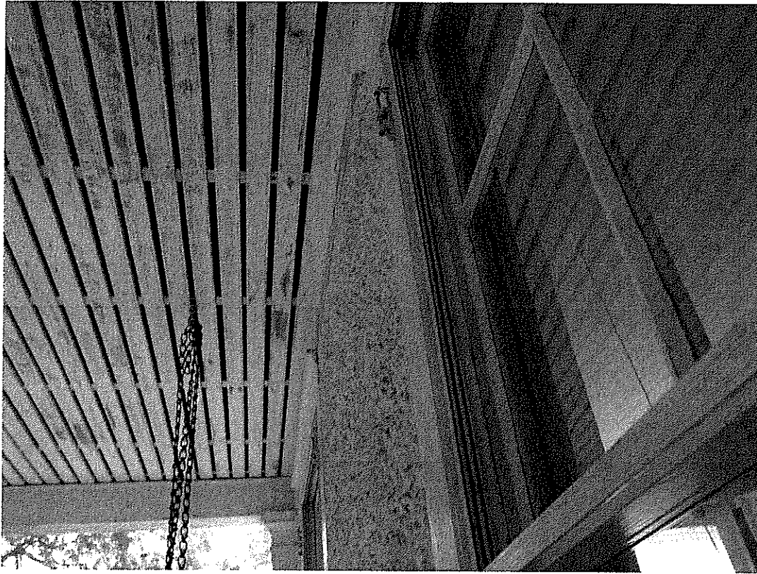
Existing triple-track storm window
