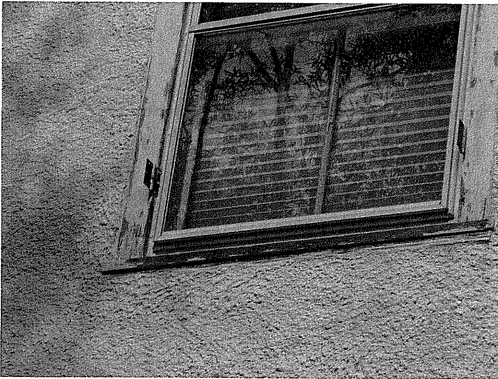
View of original window needing conservation, with existing storm window in place
