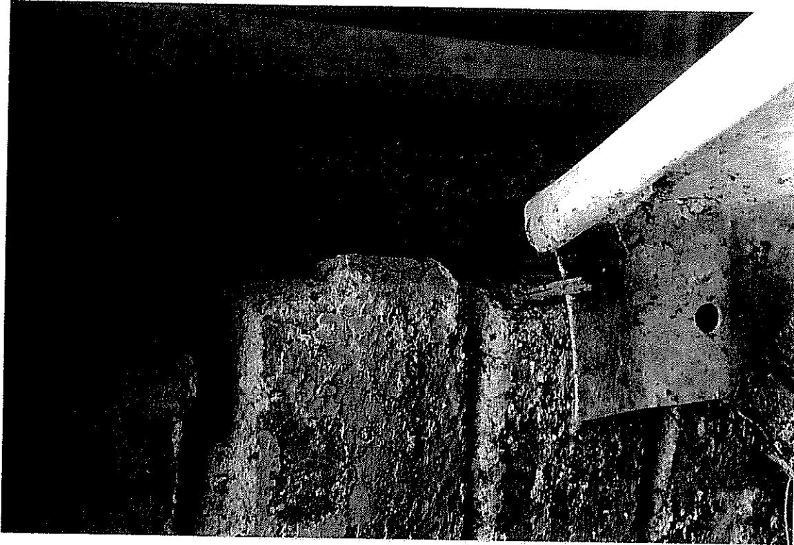
Detail: 24 Montgomery Ave., deteriorated brick foundation detail at east side window well
