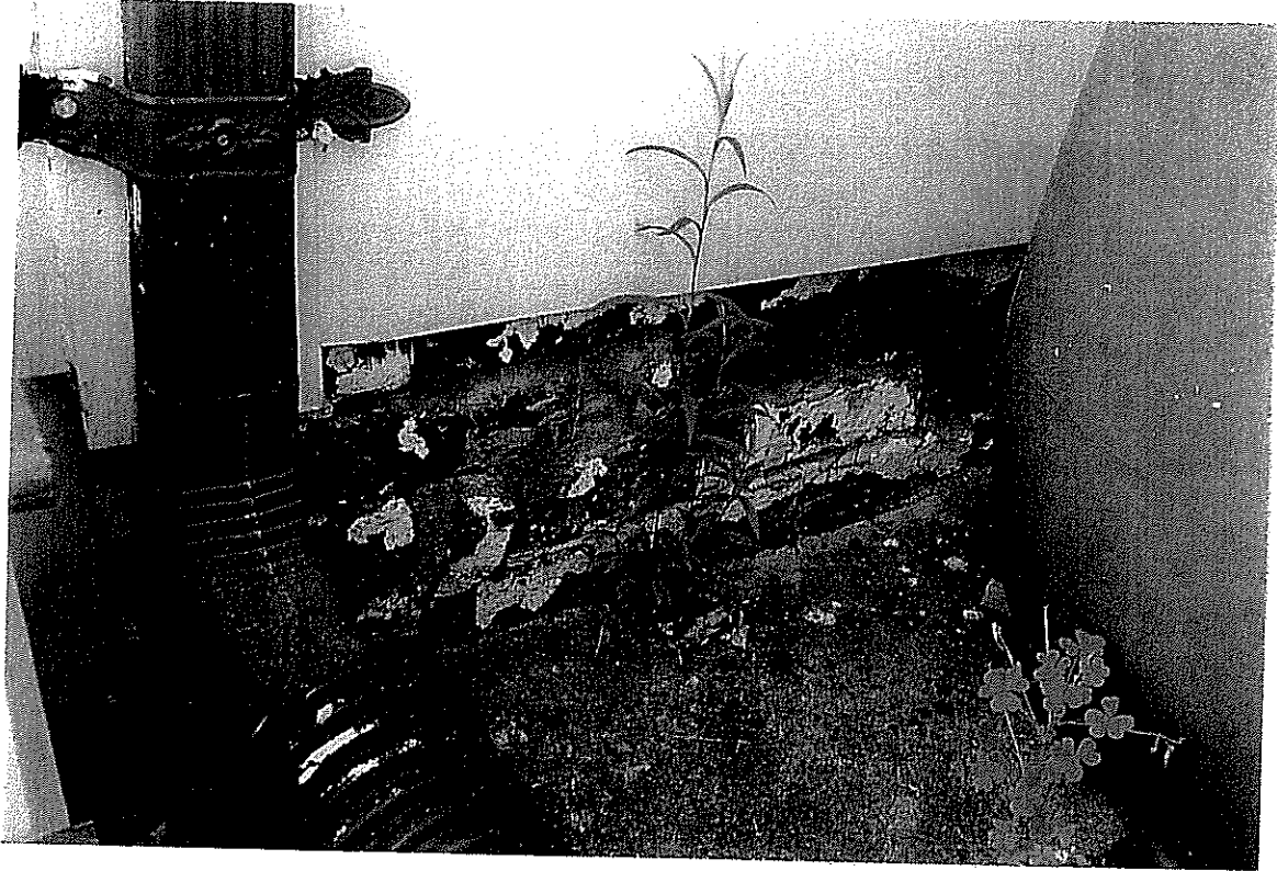
Detail: 24 Montgomery Ave., deteriorated brick foundation detail at front elevation
