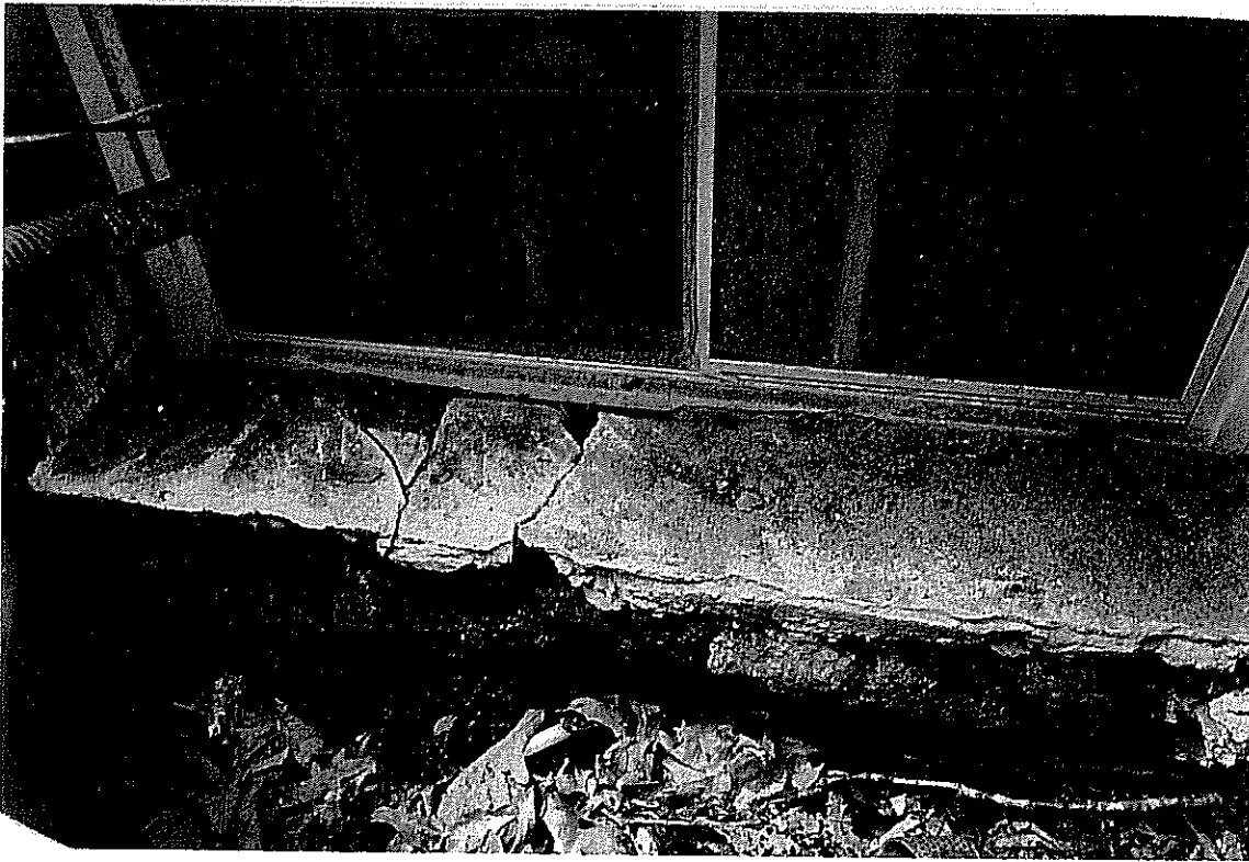
Detail: 24 Montgomery Ave., deteriorated sill detail at east side window well
