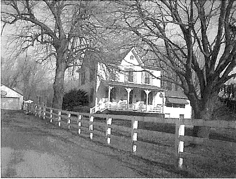
Photo 1: Boyd-Maughlin House Front (before repainting)
