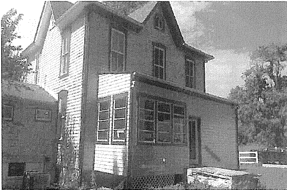
Photo 2: Rear (north) elevation showing enclosed back porch and stone stoop
