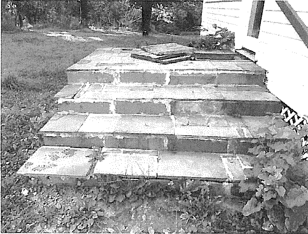
Photo 3: detail of west side of stoop with wood well cover removed
