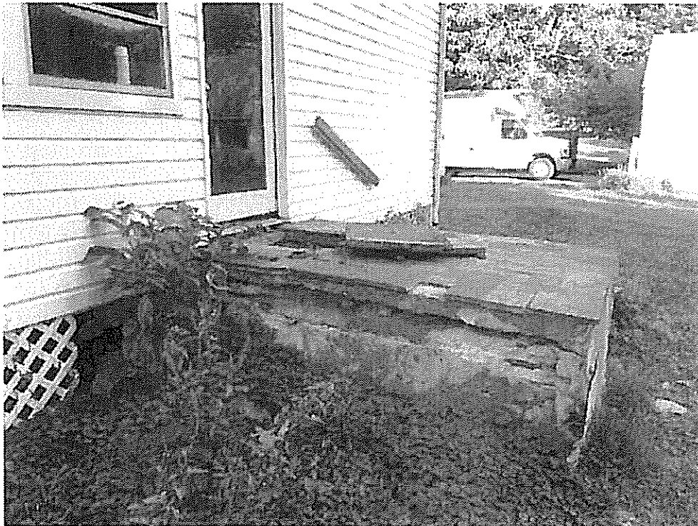
Photo 5: north side of stoop with trap door open
