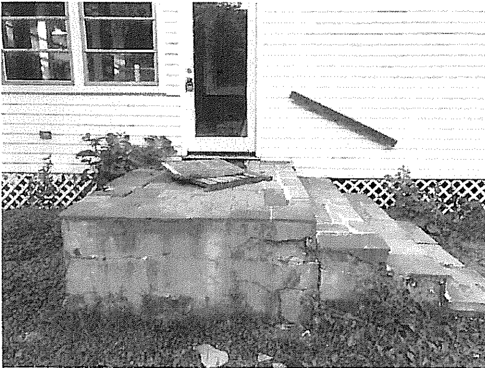
Photo 4: view of north side of stoop
