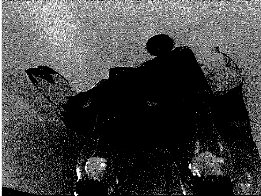
View of visible mold growth directly below second floor bathroom. IT is BEC opinion that the plumbing likely ruptured during the cooler seasons.
