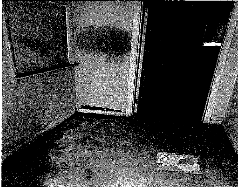
View of visible mold growth on gypsum board sheeting within the basement. In addition, visible water staining and swelling of the vinyl flooring
