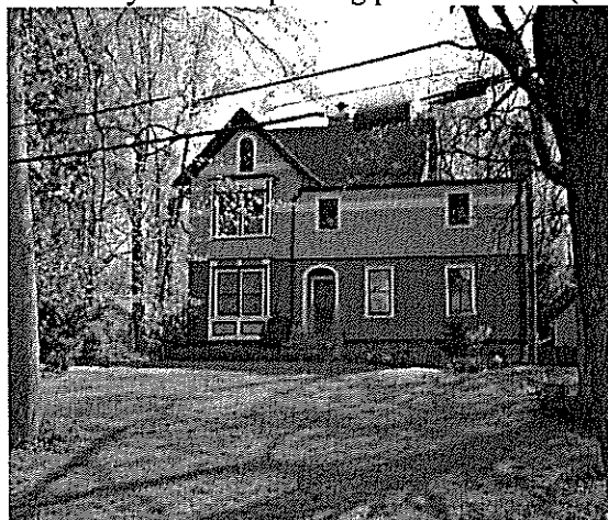
Figure 1: Pine Street (primary) facade
