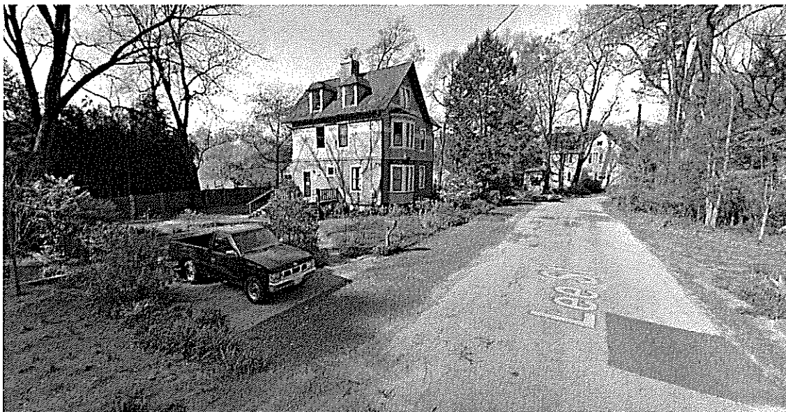
Figure 2: Lee Street elevation with existing parking pad
