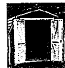
Doors are reinforced with 2" x 4" bracing.
