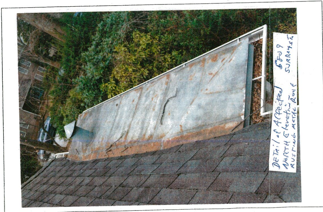
Detail: DETAIL of AFFECTED NORTH Elevation - RUSTING METAL ROOF 5809 SURREY ST.
