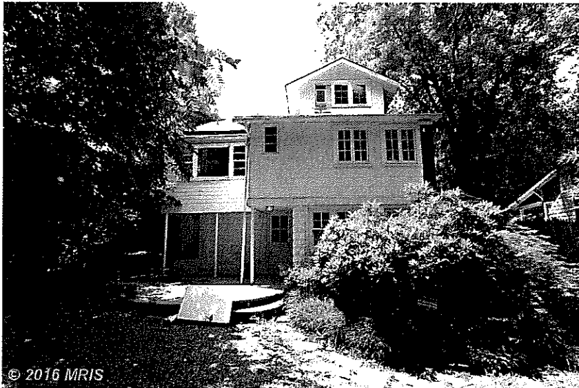
Current condition of rear of house.
