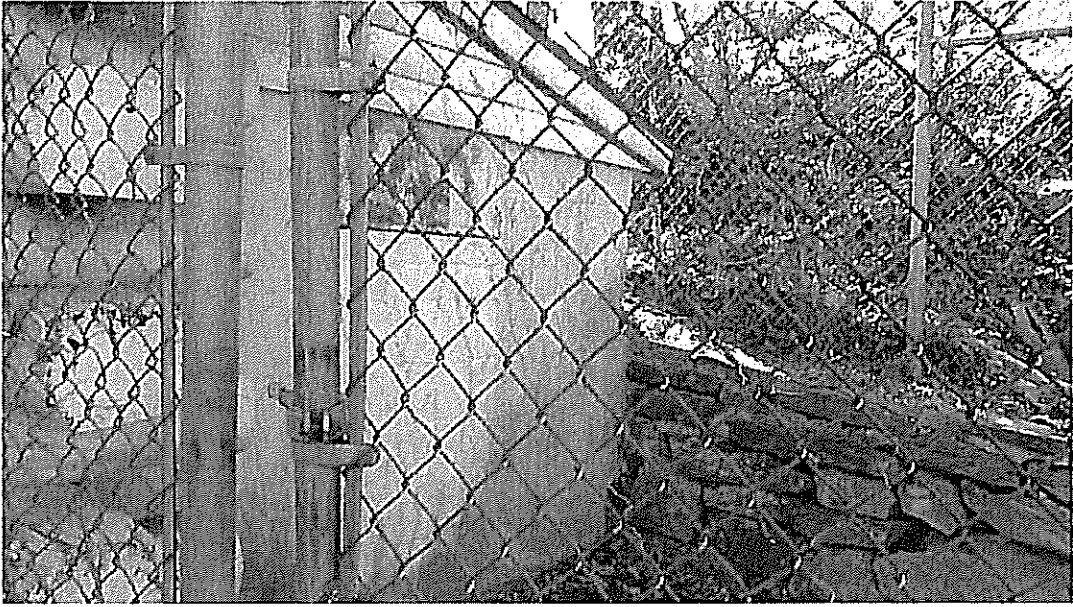
Rear Enclosed Restroom Addition
