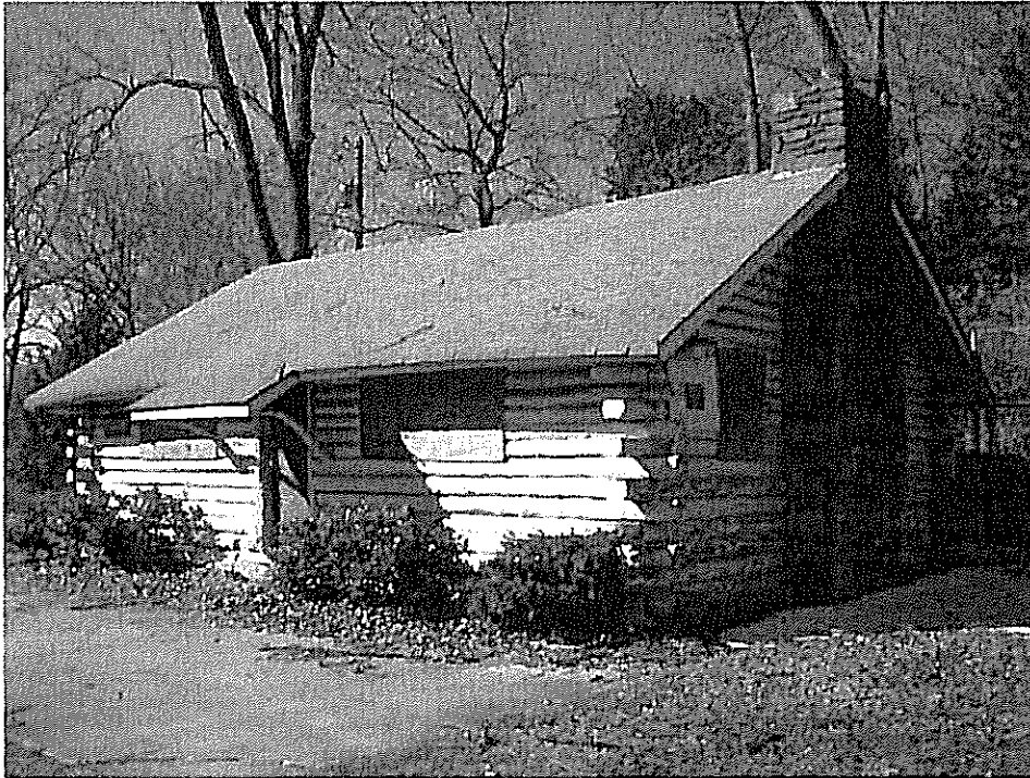
East (main) and North elevations
