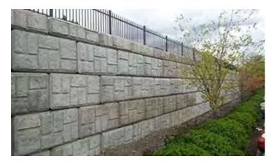
Figure 6: MSE Retaining Wall Example
