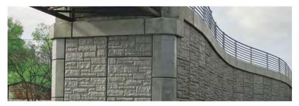
Figure 17: Ashlar Stone Abutment Example
