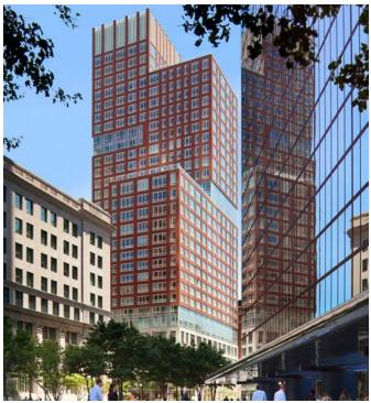
Massing broken down into smaller volumes to reduce bulk
