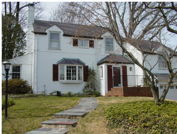
FIGURE 15b. 4700 Merivale Road M-NCPPC 3-20-2006
