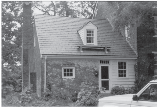
Roof replacement and dormer repair at Chiswell's Inheritance in Poolesville qualified for a County Historic Preservation tax credit.
