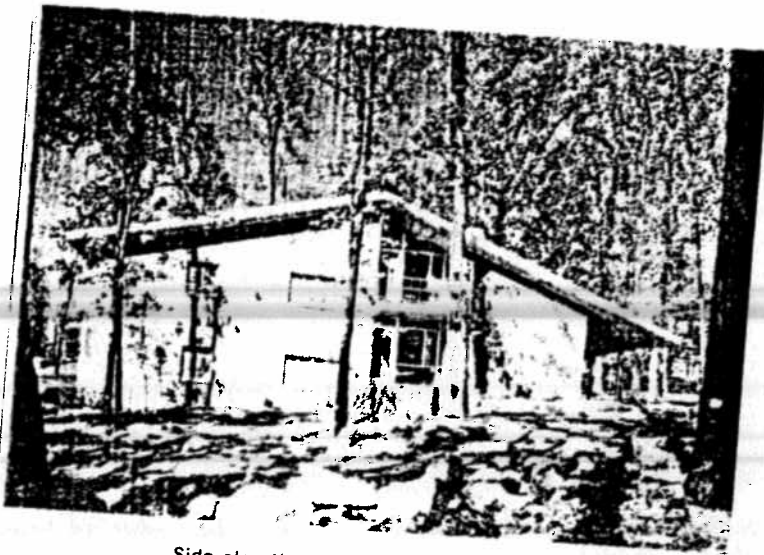
Side elevation shows how changes in levels of split match changes in the grade. Architects Keyes and Lethbridge used a contour map (which shows grades and existing trees) in developing site and house plans. Since this is the southwest side of the house windows were held to a minimum, except for balcony and terrace (see opposite).
