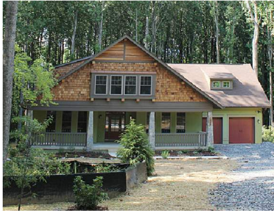
1903 BRIGHTON DAM ROAD (3,770 SF) BROOKEVILLE WOOLEN MILL AND HOUSE
