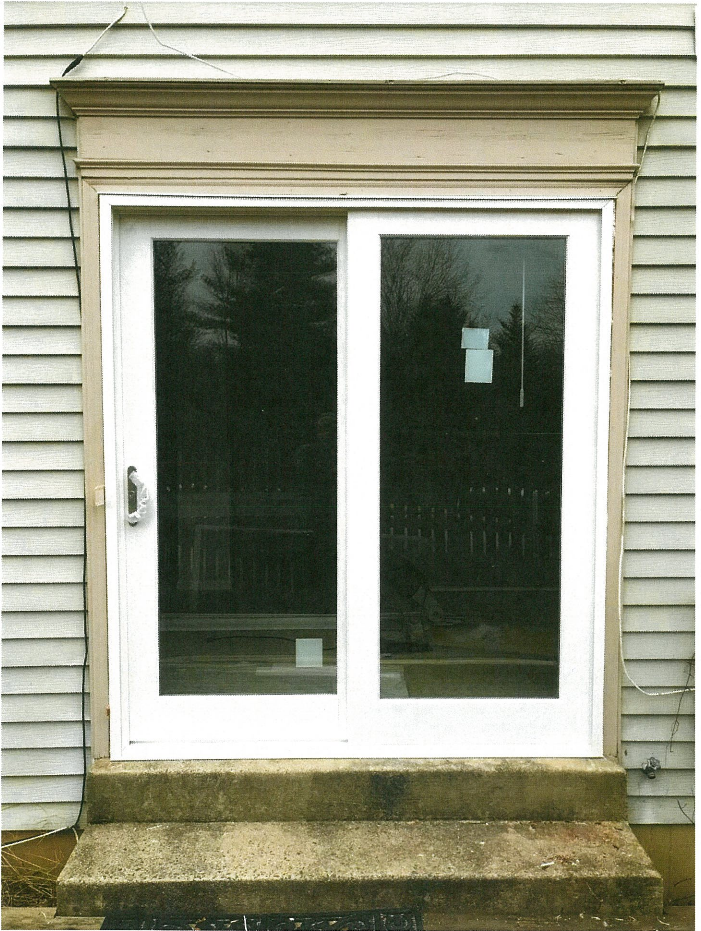
Anderson door to replace glass blocks
