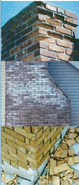
Severe spalling and deterioration is caused by water penetration.
