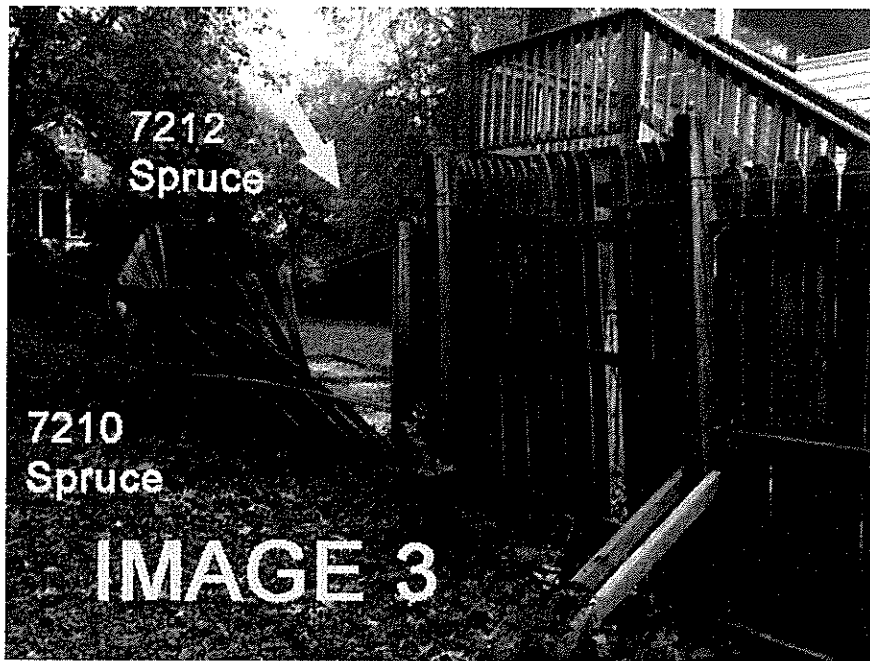
Detail: Image 3 – Collapsing portion of wood fence along the property line of 7210 Spruce and 7212 Spruce. See the diagram we provided which shows location of photo.
