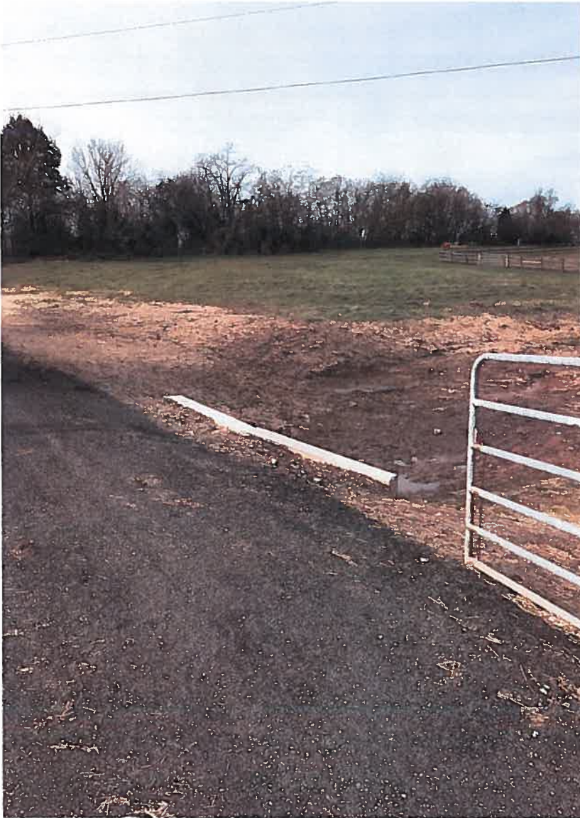
North side of the culvert (open horse gate on right). Millings to be removed and grass restored following completion of construction work. House is located beyond the photo to the upper left-hand corner.
