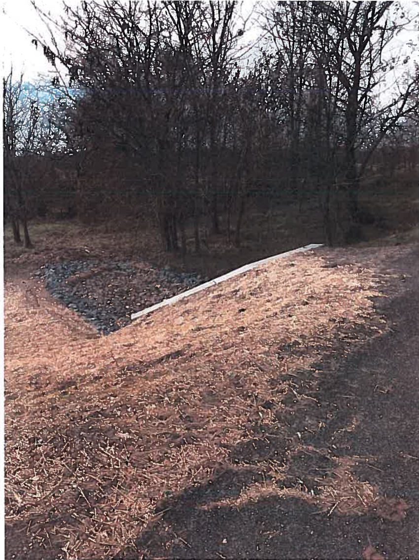
South side of the culvert showing rocks that will be covered with plantings to restore rural appearance. Millings to be removed following completion of onsite construction work.
