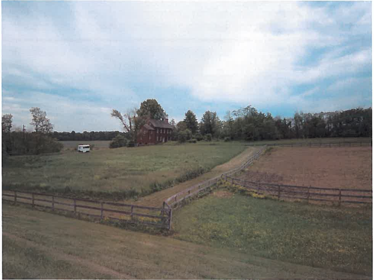
North and East elevations. Culvert is beyond the left side of the photo following the fence line. Culvert is located approximately where dot has been drawn onto the page.
