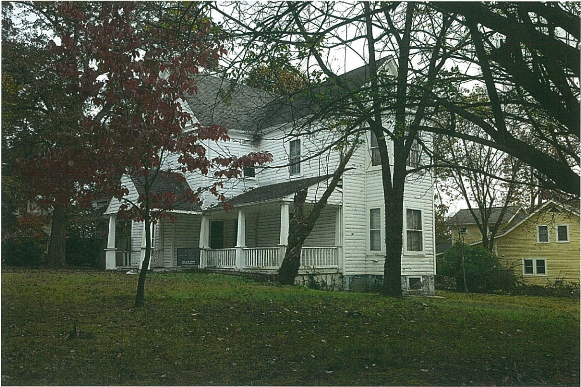
VIEW FROM INTERSECTION OF COLUMBIA & PINE AVE.
