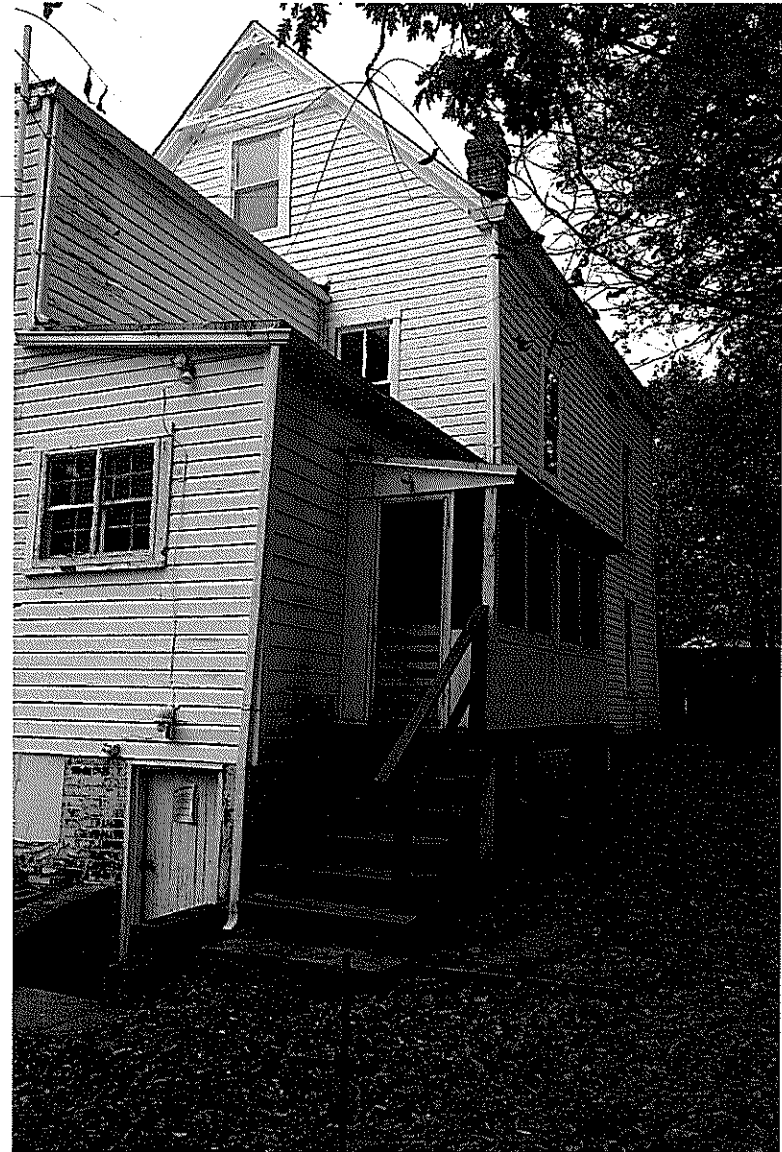
VIEW OF EXIST. SIDE SCREENED PORCH TO BE DEMOLISHED AND REPLACED W/A NEW, LARGER SCREENED PORCH.
