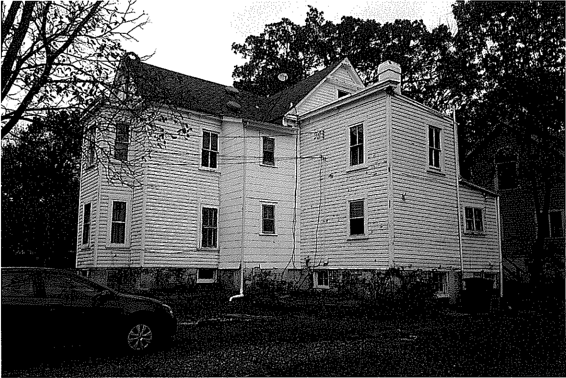
EXISTING REAR VIEW FROM PINE AVE.
