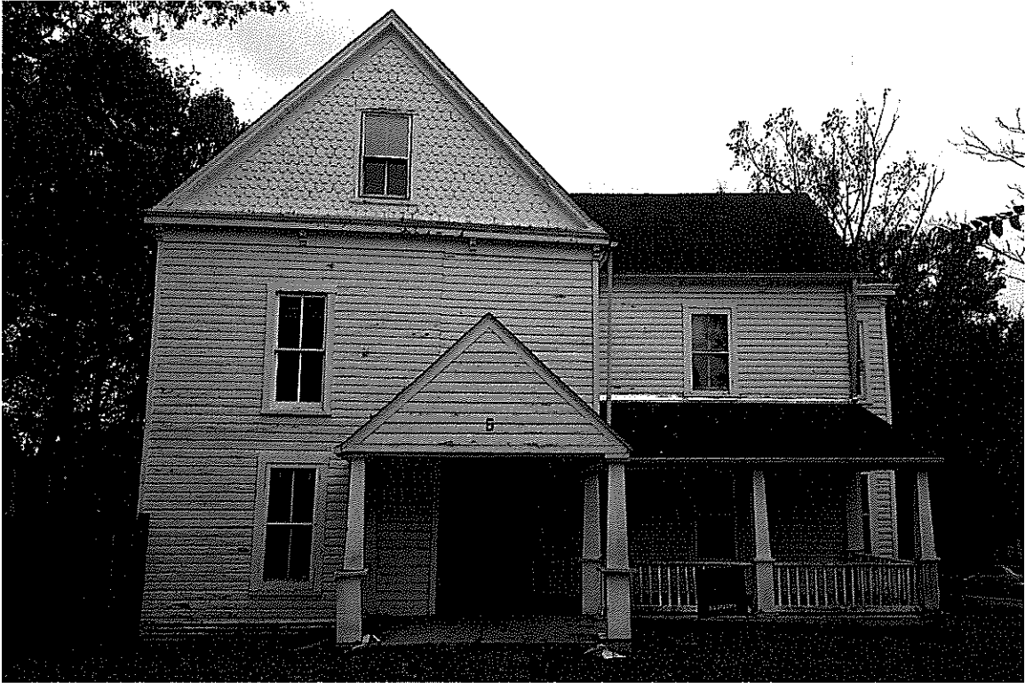
EXISTING FRONT VIEW FROM COLUMBIA AVE
