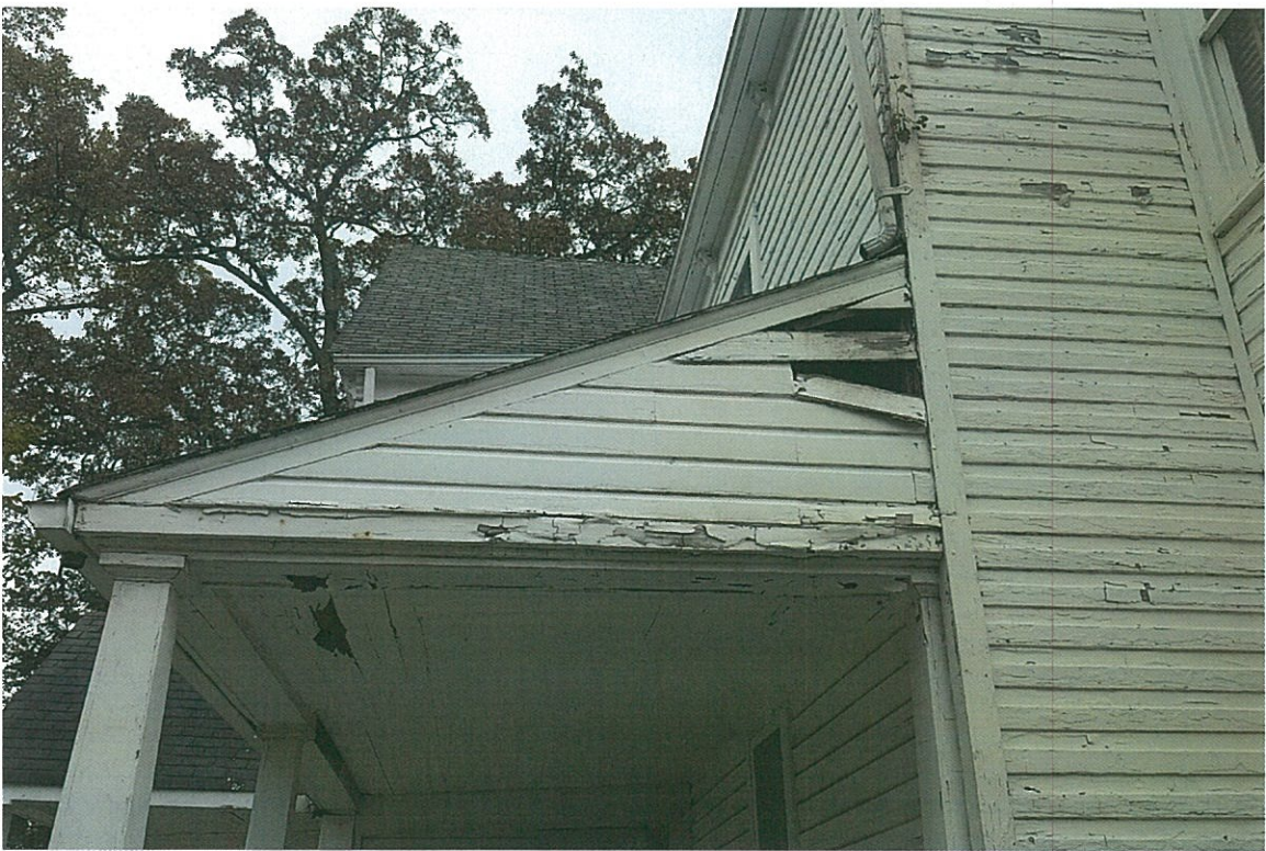
EXAMPLE OF DAMAGED SIDING
