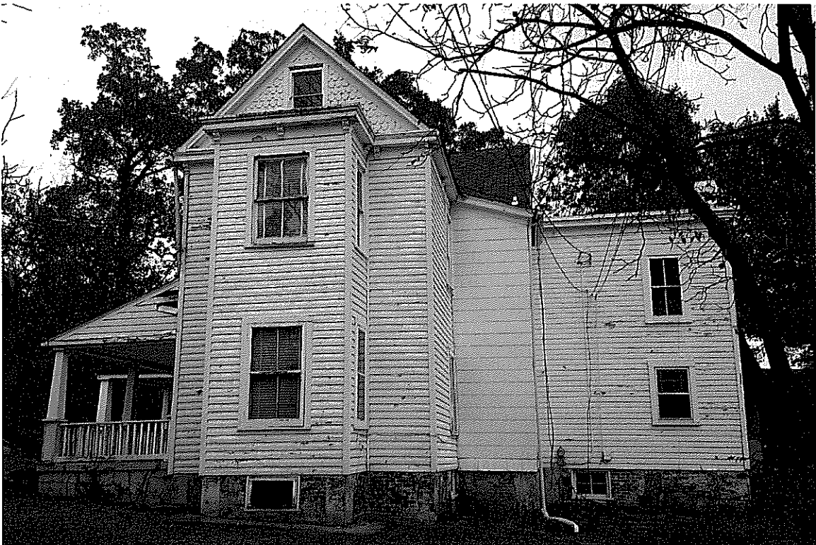
EXISTING SIDE VIEW FROM PINE AVE.
