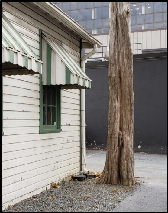
Figure 17 – Southeast Corner of Building
