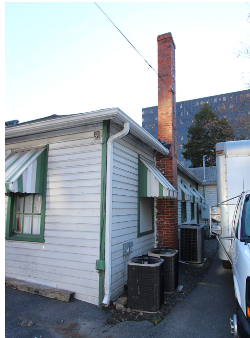
FIGURE 28 North side of west elevation including brick chimney and condenser units.
