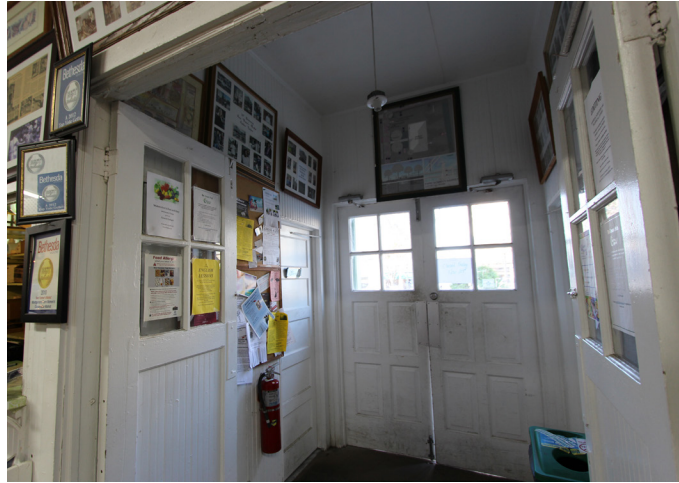
FIGURE 61 Interior of vestibule looking west. Traceries.
