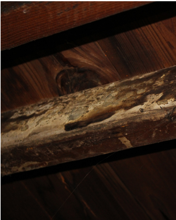
FIGURE 82 Termite damage evident in attic.
