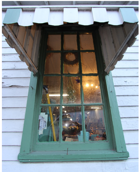
FIGURE 21 Original twelve-light, wood-sash pivot window.
