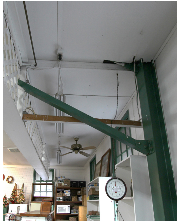
FIGURE 77 Original structural steel beams and braces visible along the west and east walls.
