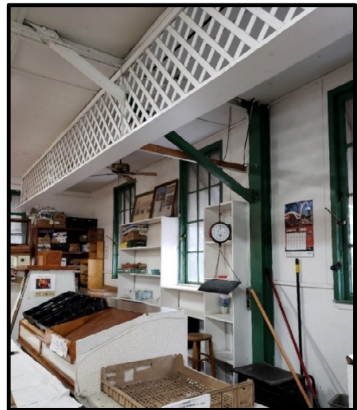
Figure 11 – Typical Steel Column and Kicker
