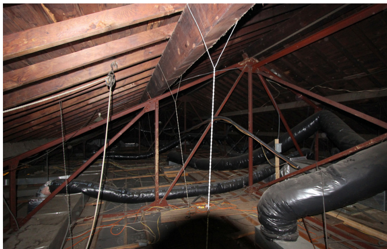
FIGURE 78 Attic, roof trusses, and contemporary mechanical equipment, looking north.
