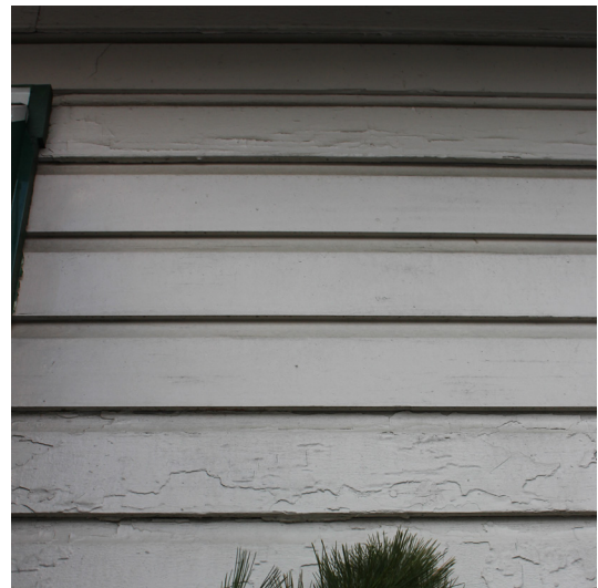
FIGURE 35 Replacement siding visible on east elevation.
