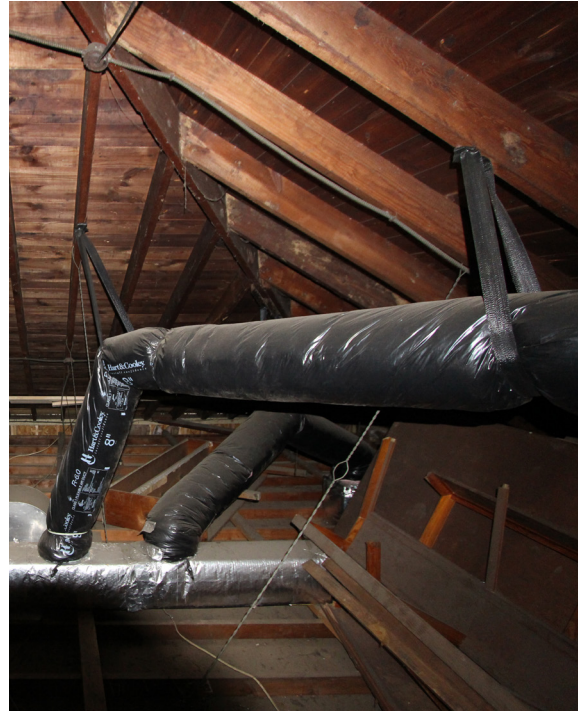
FIGURE 81 Wires supporting non-original ceiling joists.
