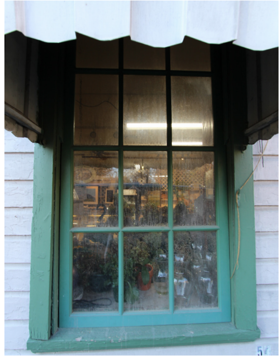
FIGURE 45 Replacement window on the east elevation.
