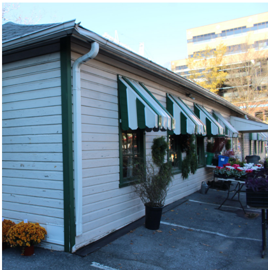
FIGURE 34 Reconstructed southeast corner.
