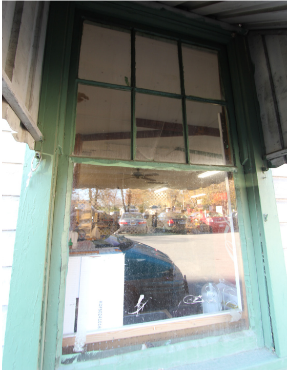
FIGURE 44 Extant window missing lower muntins.
