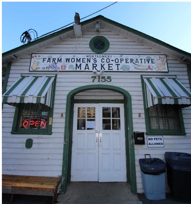
FIGURE 24 Replacement doors at front entrance.
