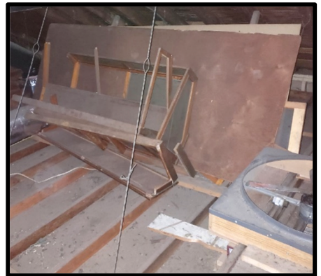
Figure 14 – Stored Items on Ceiling Framing
