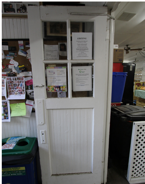
FIGURE 71 Detail of door accessing market space from vestibule.
