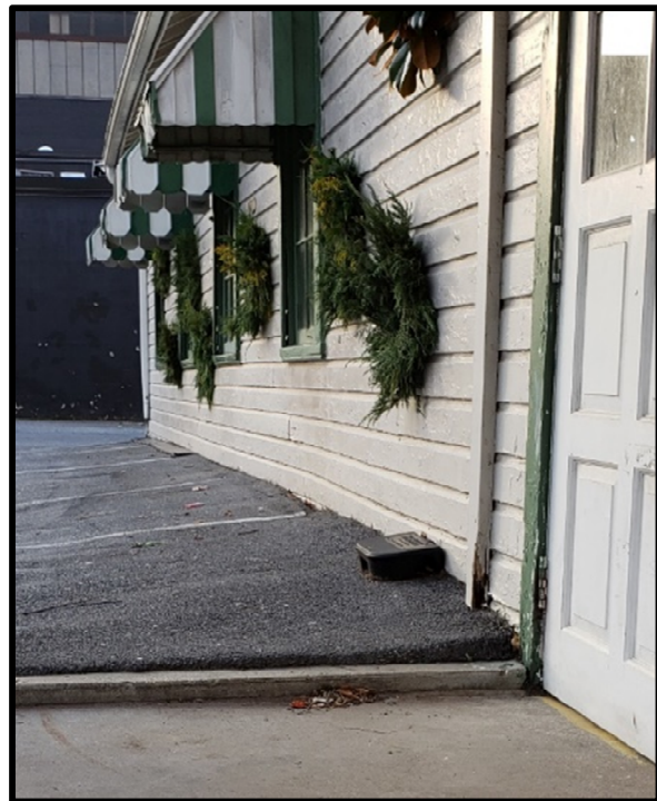
Figure 4 – Built Up Asphalt Against East Wall
