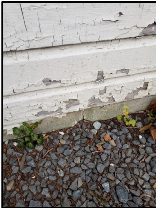
Figure 3 - Existing Drainage Conditions Along East Wall
