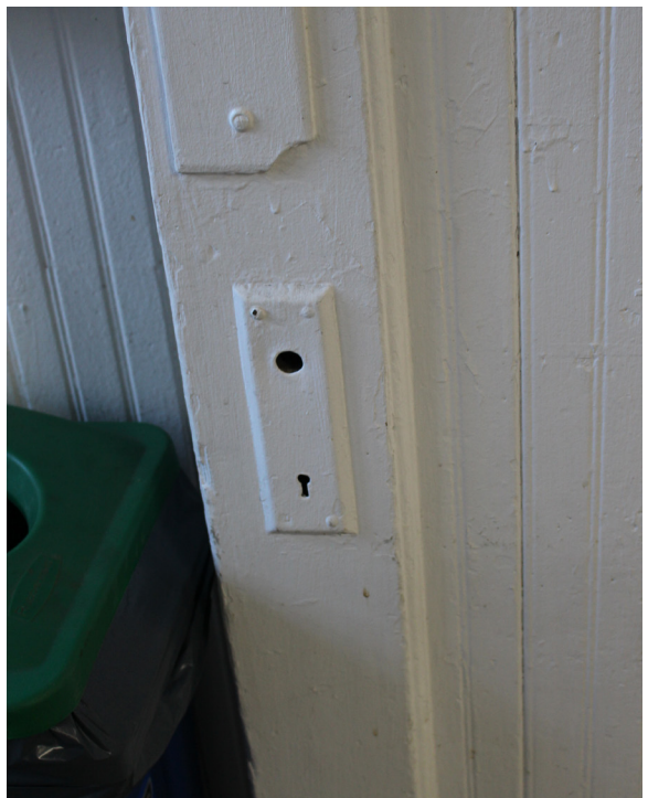
FIGURE 70 Detail of painted original hardware.
