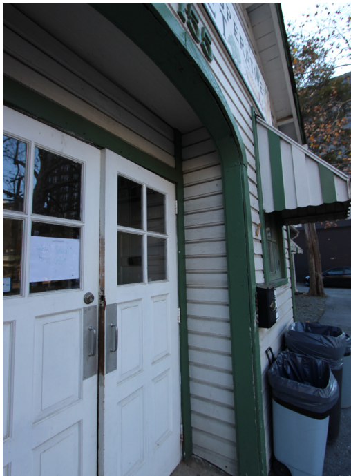
FIGURE 27 Contemporary entry doors and interior of front projecting pavilion.
