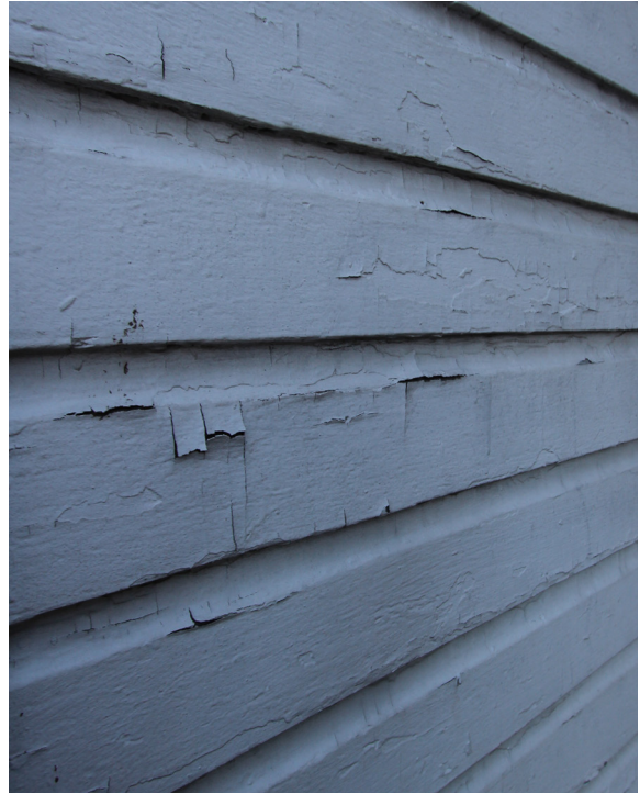
FIGURE 19 Detail of the wood siding and deteriorated paint.
