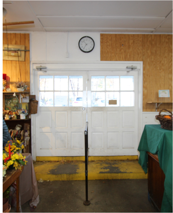
FIGURE 73 Interior view of east elevation door and concrete step.
