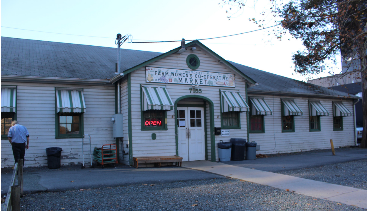
FIGURE 22 Facade looking southeast.
