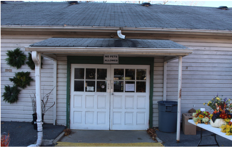
FIGURE 30 Non original rear doorway
