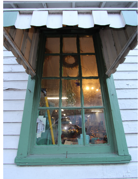
FIGURE 43 Extant original wood windows.
