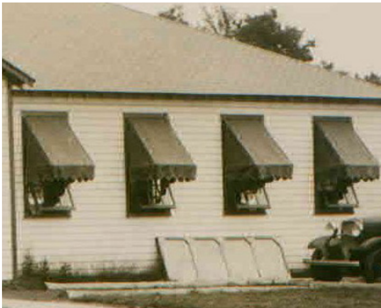
FIGURE 42 Detail of pivoting wood-sash windows, c. 1930s. Montgomery County Historical Society.
