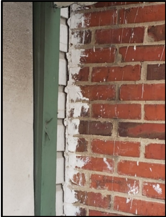
Figure 16 – Visible Gap Between Buildings and Chimney
