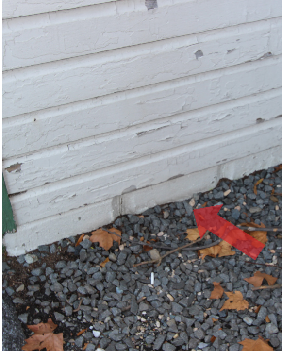
FIGURE 18 Siding and exposed concrete block foundation stem wall (identified with arrow) along the west elevation.
