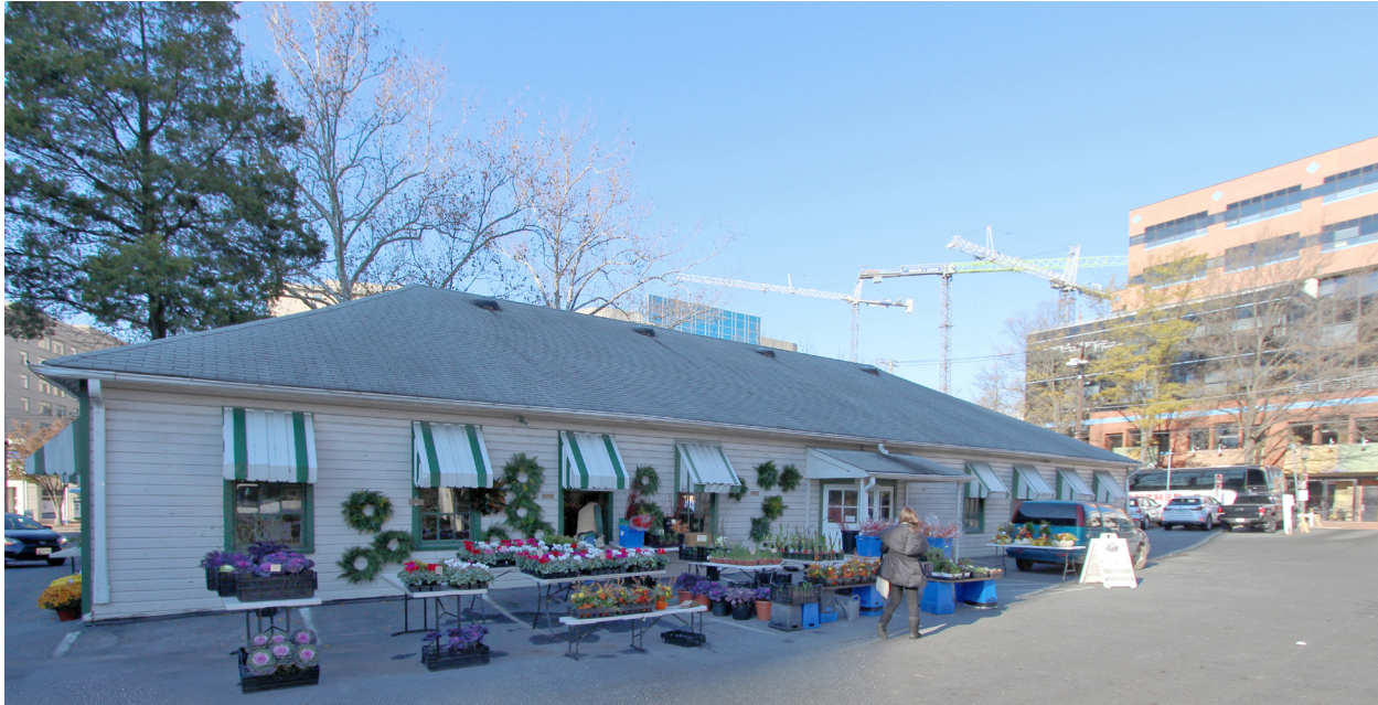
FIGURE 48 View of east elevation, roof and contemporary roof venting, looking west.
