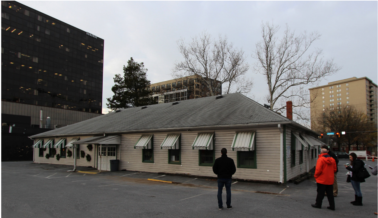
FIGURE 29 Rear elevation, looking southwest. Tracerics.
