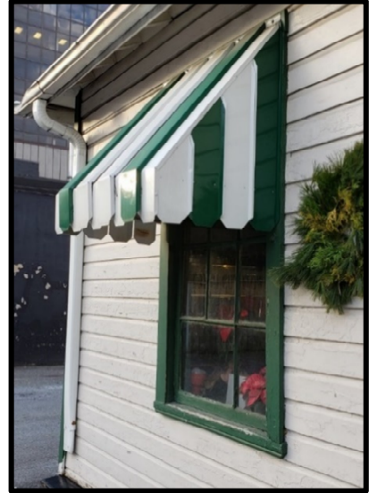
Figure 12 – Cold formed Steel Awnings
