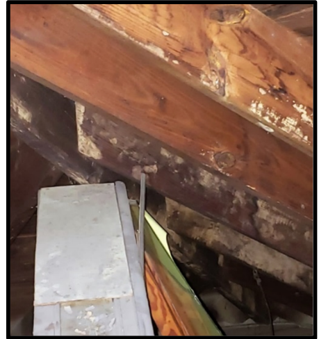
Figure 13 – Southeast Roof Framing
