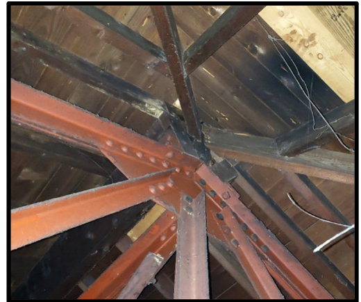
Figure 10 – Hip Connection
