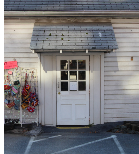
FIGURE 41 North elevation doorway and pitch roof.
