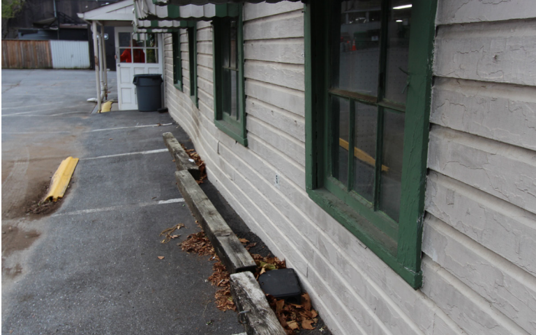
FIGURE 32 Undulation of the elevation
