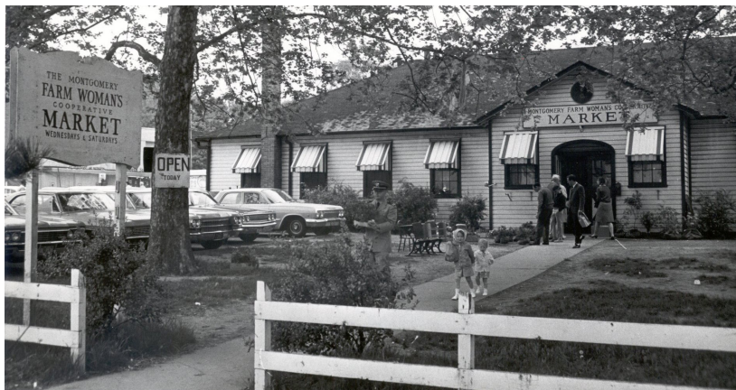
FIGURE 53 Deteriorated lawn, mature trees, and foundation plantings, 1968. Montgomery County Historical Society.
