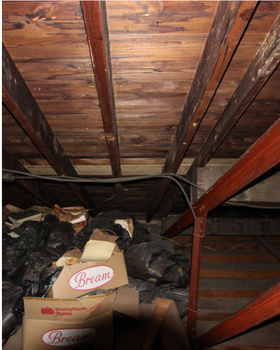
FIGURE 80 Attic truss and roof structure, looking east.
