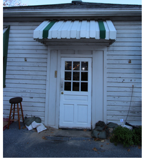
FIGURE 39 South elevation doorway and sandbags.
