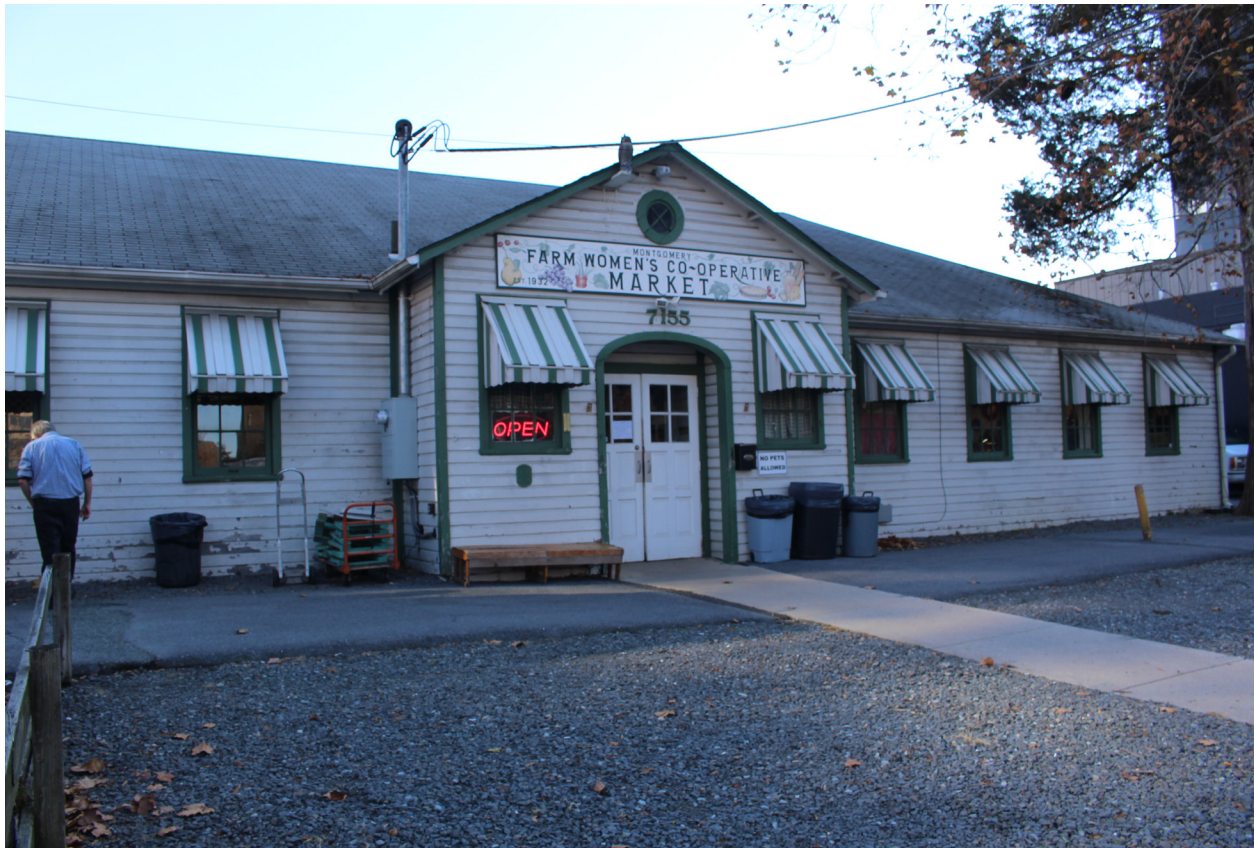
FIGURE 01 West (front) elevation of the Farm Women's Market. EHT Tracerics, 2018.
