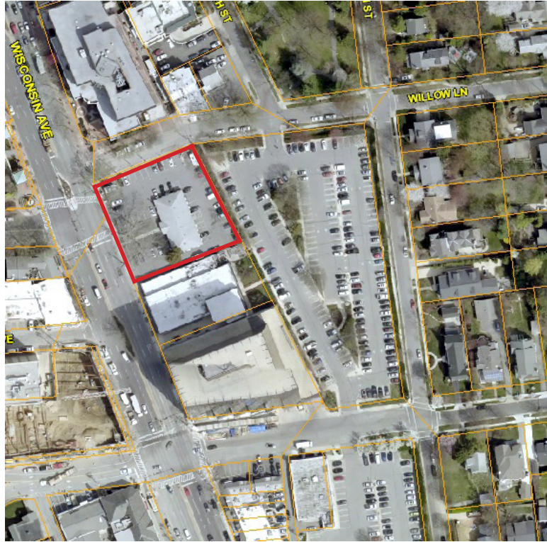
FIGURE 02 Aerial photograph of site; Farm Women's Market parcel outlined in red. Montgomery County Index of Record Plats, Montgomery Planning.
