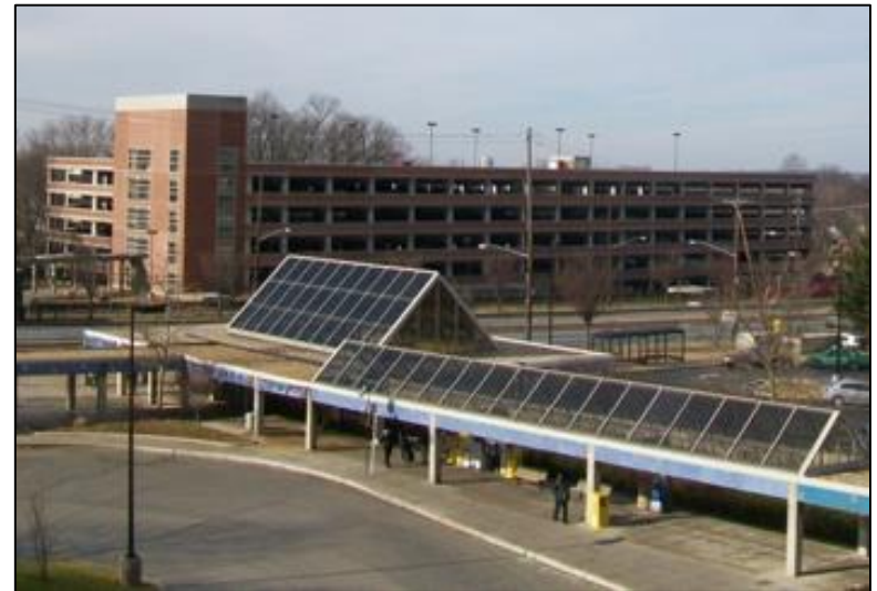
Glenmont Metro Station 1200 space parking garage.
