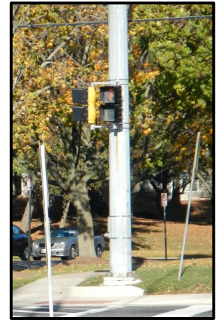
Figure 10: Countdown Pedestrian Signal
