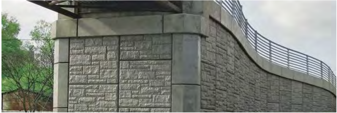
Figure 17: Ashlar Stone Abutment Example
