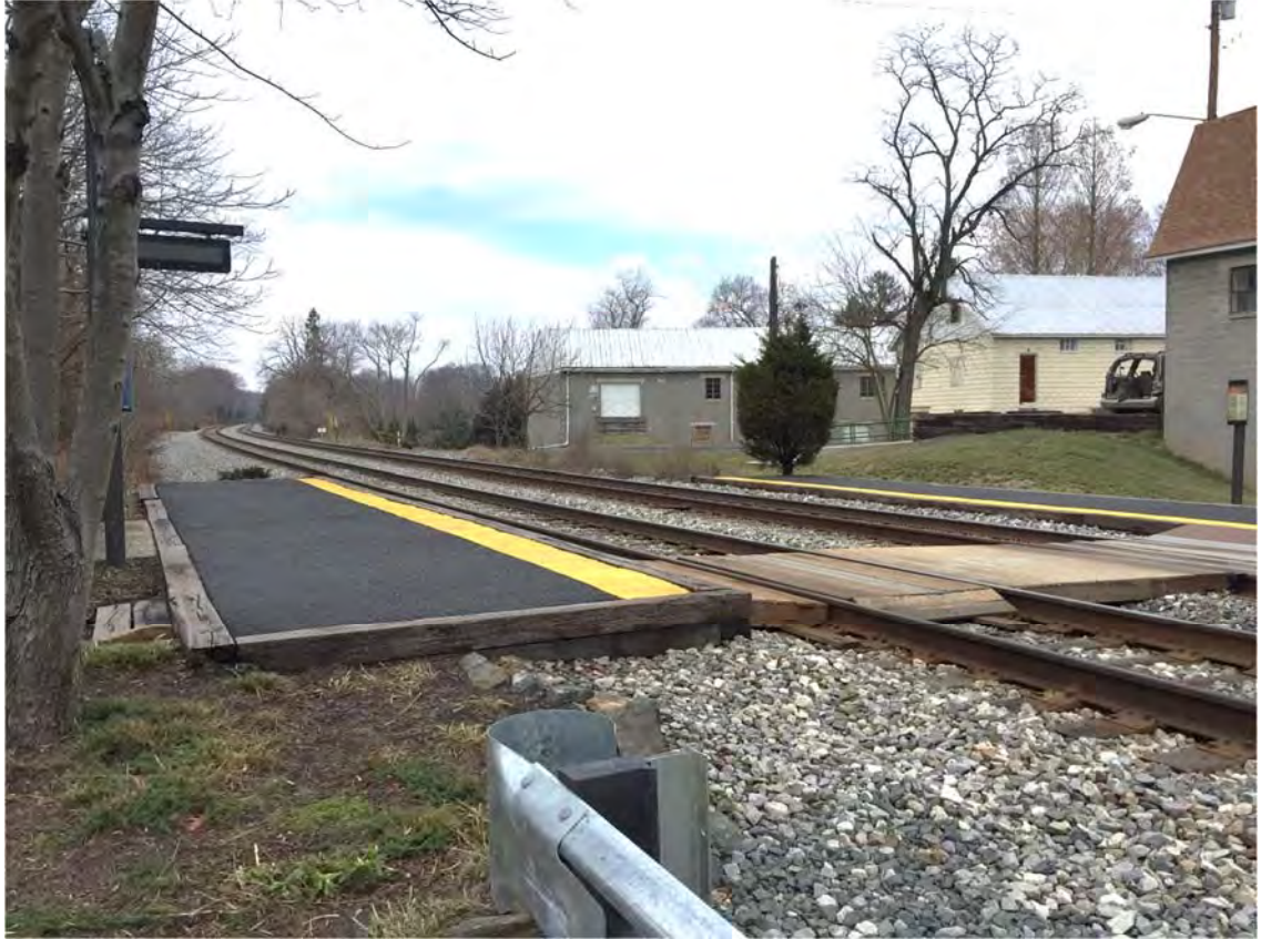
Figure 2: MARC Station Platform (looking west)
