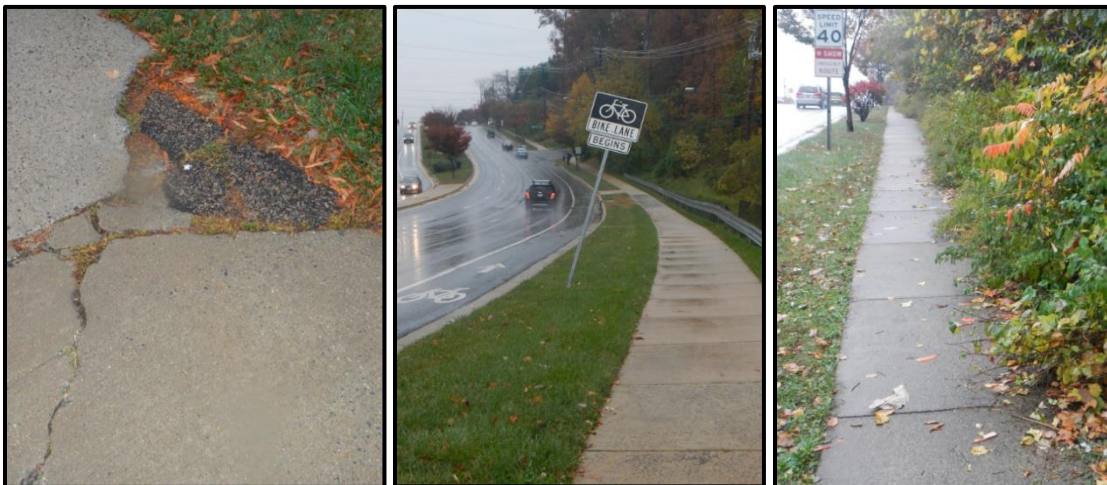
Left: Damaged sidewalk on the south side of Middlebrook Road. Center: Sign is leaning east of Great Seneca Highway. Right: Overgrown vegetation greatly reduces sidewalk width.
