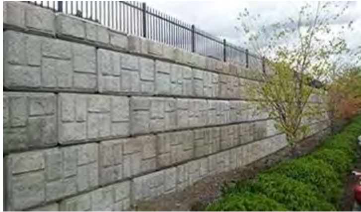
Figure 6: MSE Retaining Wall Example
