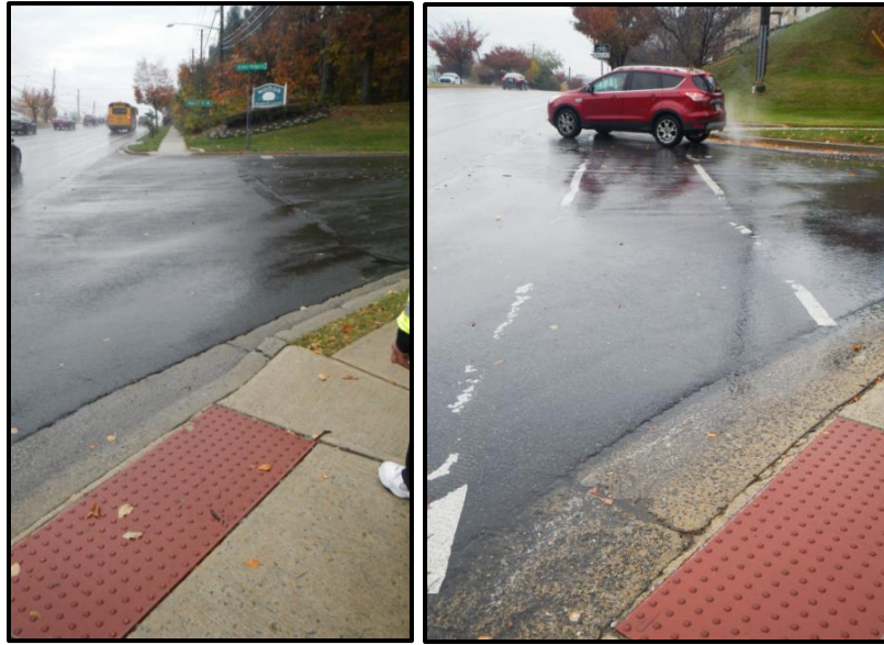
Left: No marked crosswalks across side streets. Right: Crosswalk markings are faded.
