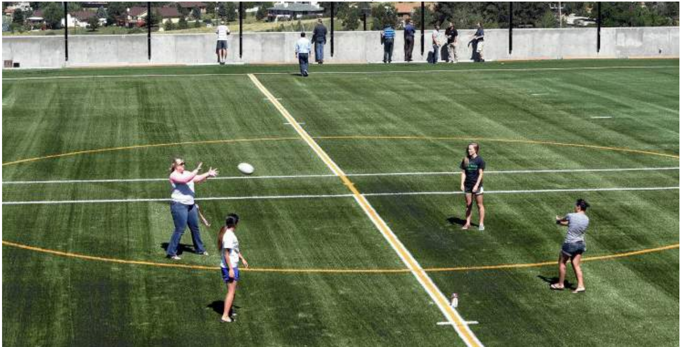
Recreational field over a parking garage.
