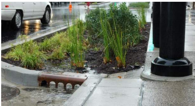
Tree planters used for stormwater retention and infiltration
