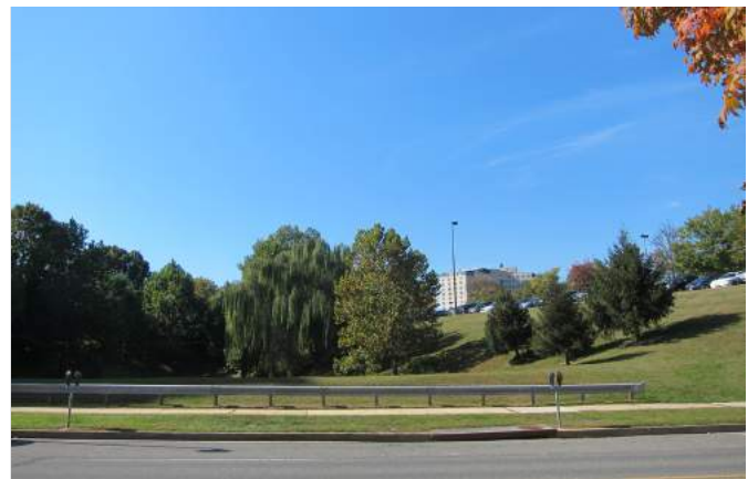
Existing stormwater pond at the Metro Site
