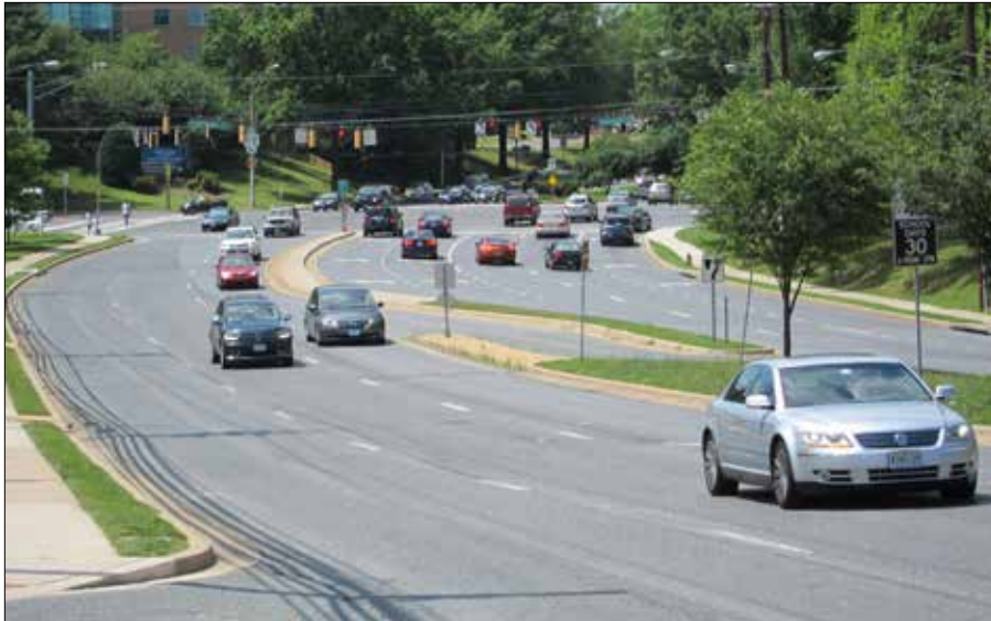
Sidewalks along Middlebrook Road in Germantown
