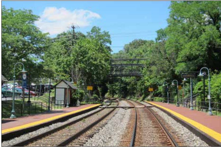
Germantown MARC Station and pedestrian bridge
