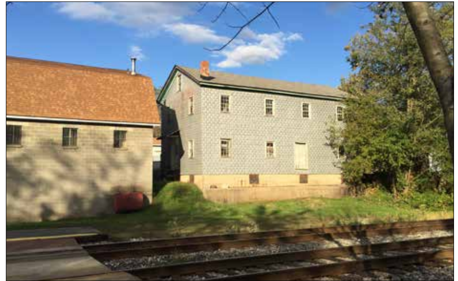
Historic Hoyle's Mill (right building)
