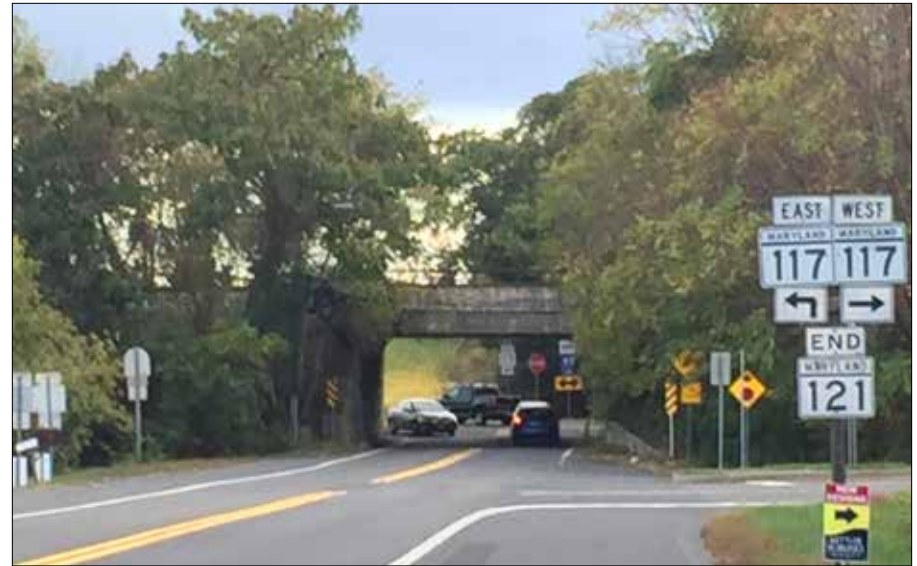
Existing underpass beneath railroad tracks in Boyds
